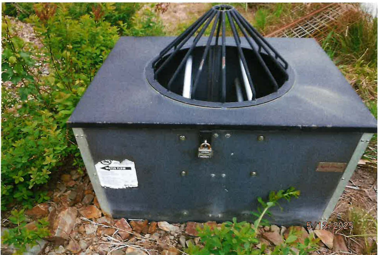
SECONDARY "WEST PIPE" AGRIDRAIN FENCED INFLOW (SLOUGH SIDE) WITH 24-INCH CULVERT INSTALLED WITH DIRECT CONNECTION TO THE COEUR D'ALENE RIVER
