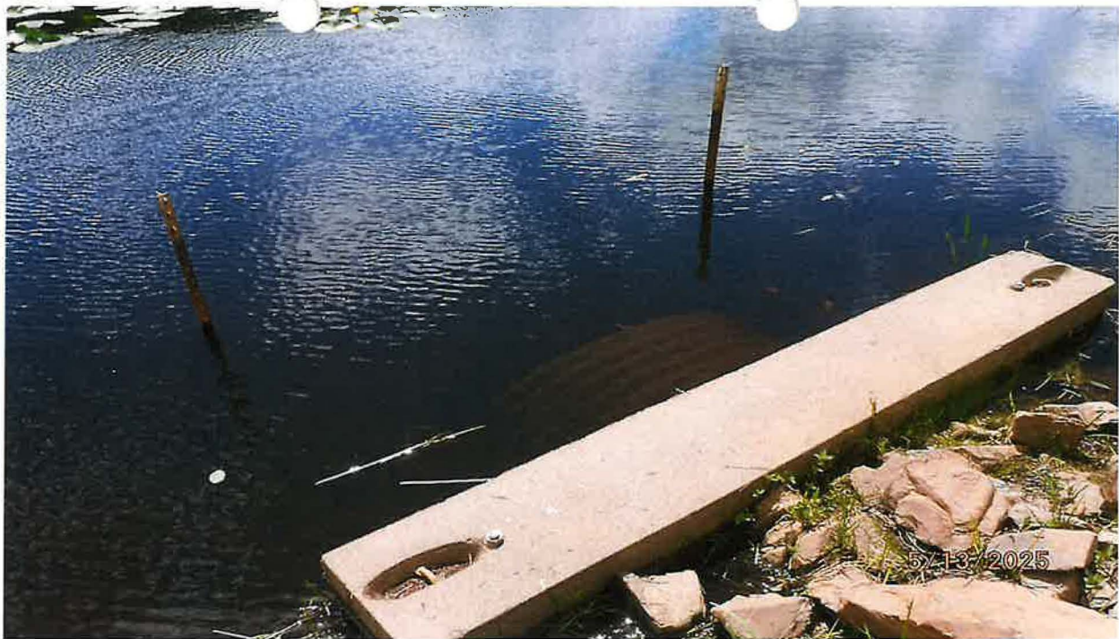
POD 1: BULL RUN CREEK SOURCE 42-INCH CULVERT WITH CONCRECT COLLAR SET TO ELEVATION 2127.75 FT (REF CONSTRUCTION CAD SCHEMATICS)
