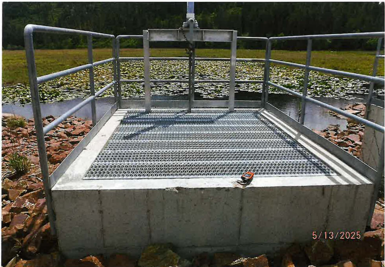
POD 1: WATER CONTROL STRUCTURE – CONCRETE SHAFT WITH SLIDE GATE AND STOPLOGS INSTALLED WITHIN GATE STRUCTURE. POD 2: SAME DEVELOPMENT AS POD 1.
