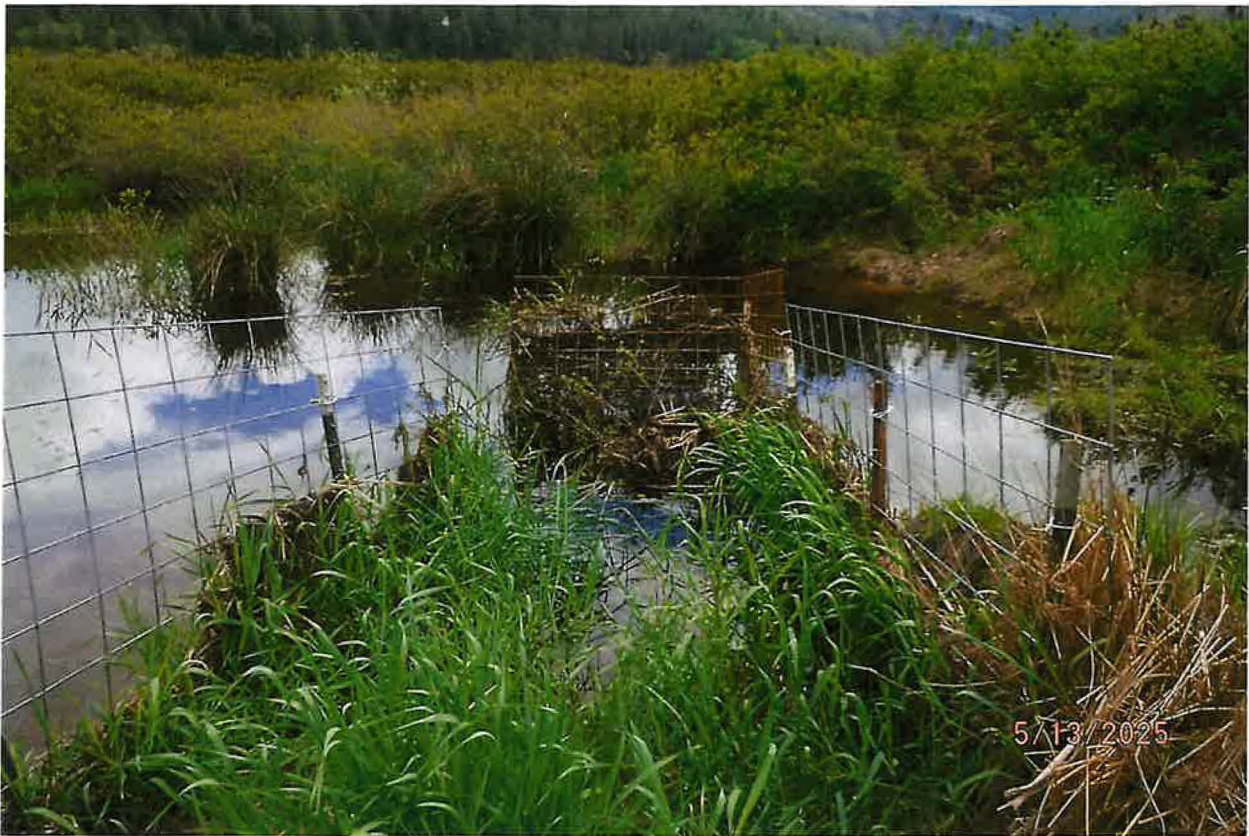
SECONDARY "WEST PIPE" AGRIDRAIN FENCED INFLOW (SLOUGH SIDE) WITH 24-INCH CULVERT INSTALLED WITH DIRECT CONNECTION TO THE COEUR D'ALENE RIVER
