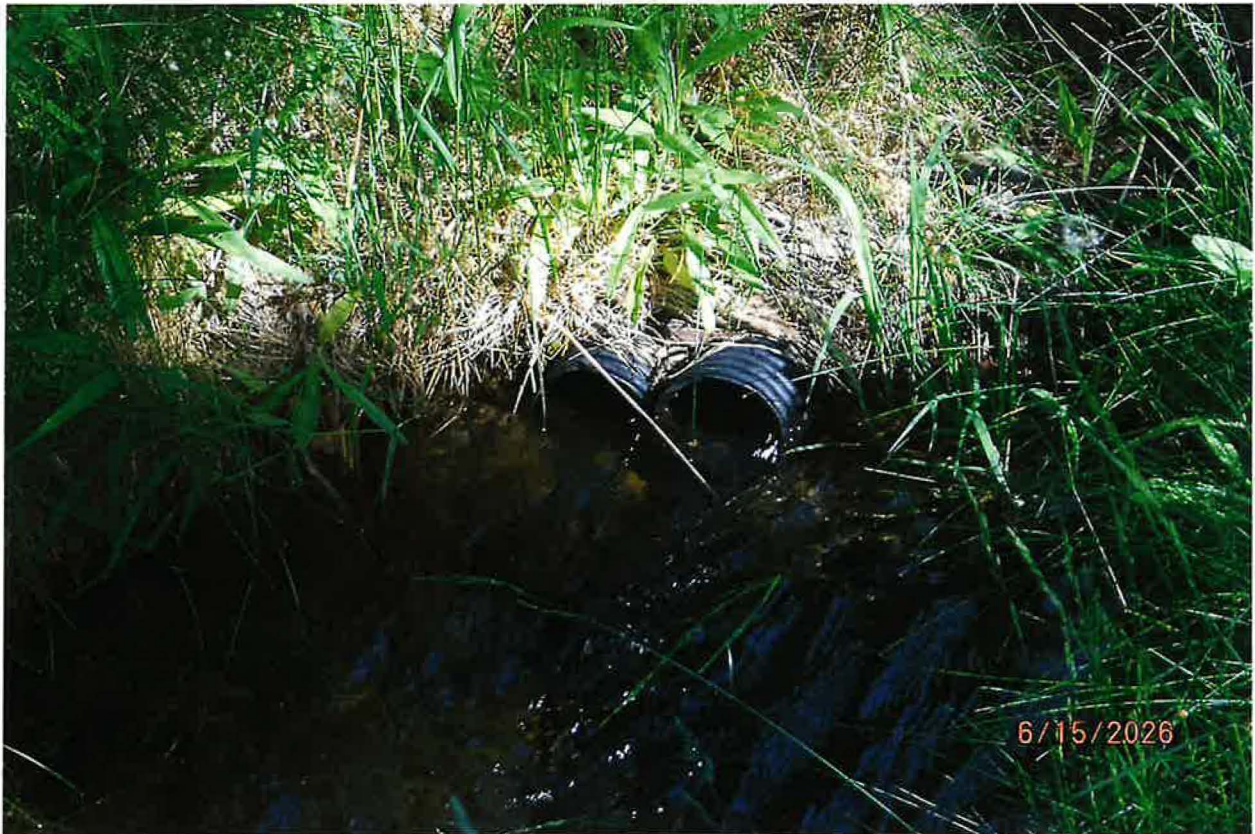
SEDIMENT BASIN PRIOR TO STORAGE POND – TWO CONVEYANCE PIPES DAYLIGHT IN A SMALL POOL BEFORE TRANSITIONING TO A SINGLE 8-INCH CORRUGATED PIPE TO POND.
