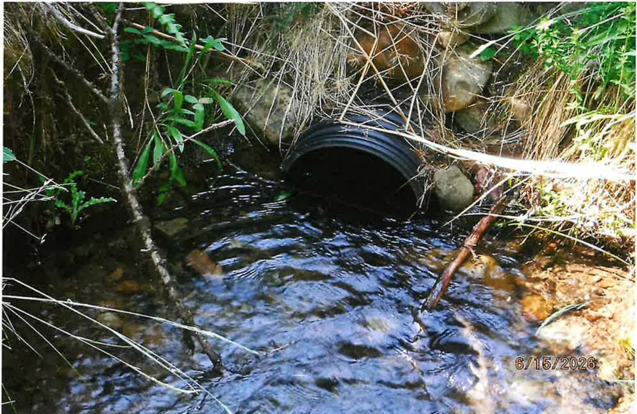
SEDIMENT BASIN – SHORT RUN OF 8-INCH CORRUGATED PIPE CONVEYS WATER TO STORAGE POND INFLOW
