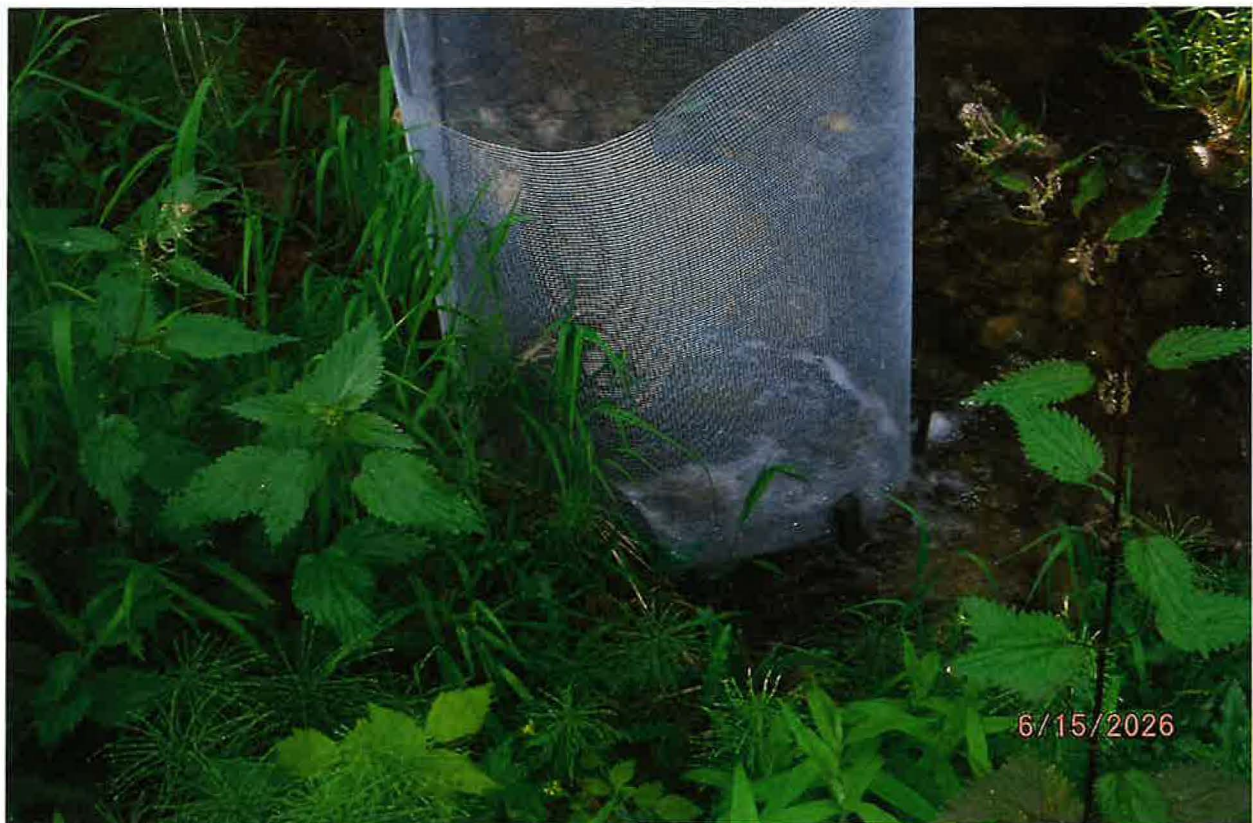
LOW SIDE OF EARTHEN DAM – OVERFLOW DISCHARGE PIPE ROUTES BY SHORT CHANNEL BACK TO MEADOW CREEK
