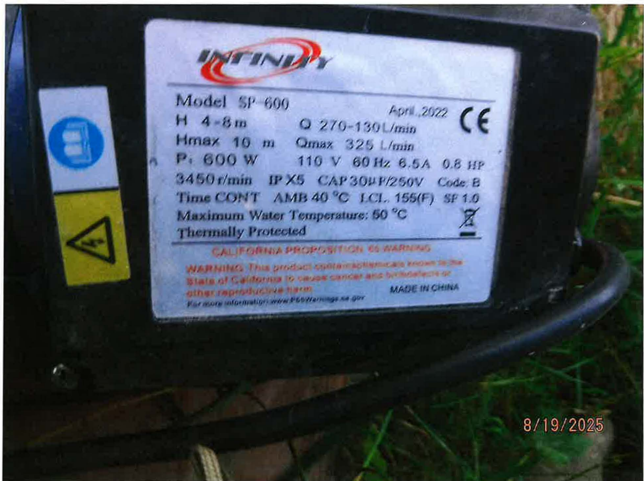
0.8 HP CENTRIFUGAL DIVERSION TO STORAGE (ASSISTS GRAVITY FLOW) INFINITY BRAND MODEL SP-600 PUMP
