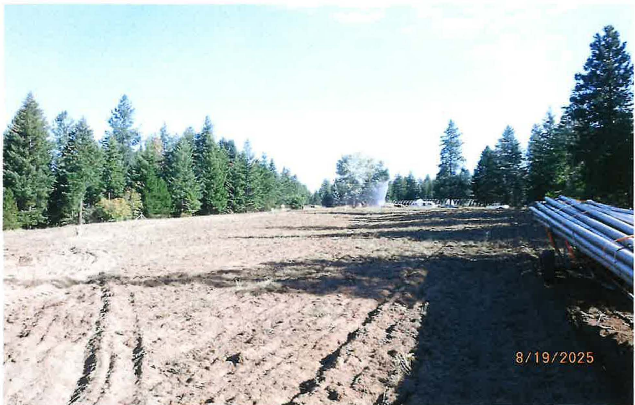
HANDLINE USED FROM SOUTHERN MOST RISER CONNECTION TO EXTEND IRRIGATION BY HANDLINE SPRINKLER ON SOUTHERN MOST FIELD OF POU
