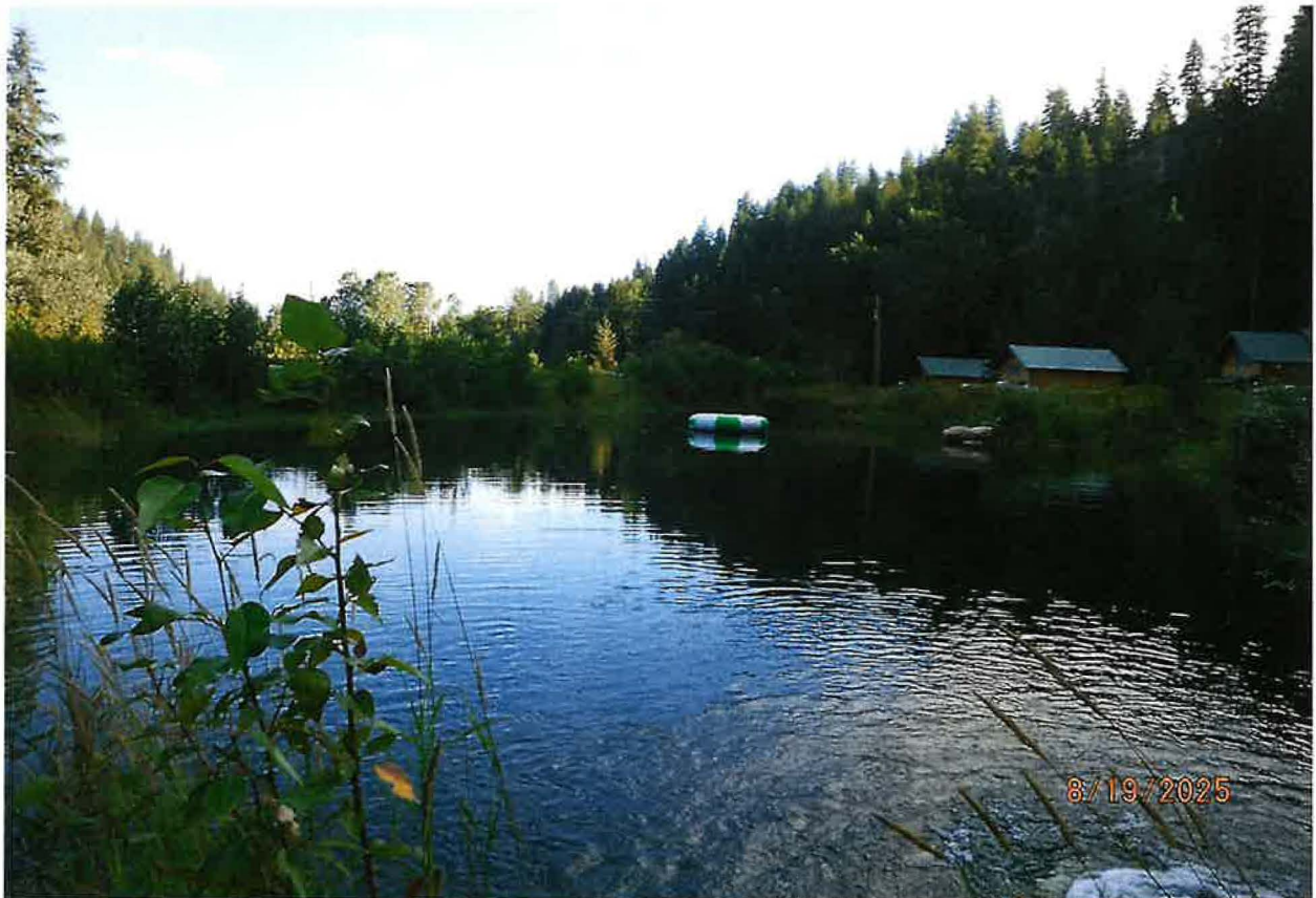
POU – IRRIGATION STORAGE AND FIRE PROTECTION STORAGE POND
