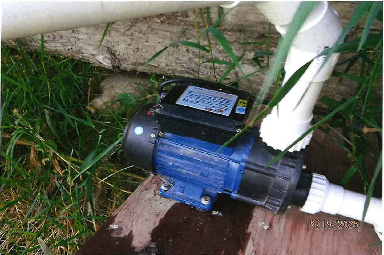
0.8 HP CENTRIFUGAL DIVERSION TO STORAGE (ASSISTS GRAVITY FLOW) INFINITY BRAND MODEL SP-600 PUMP
