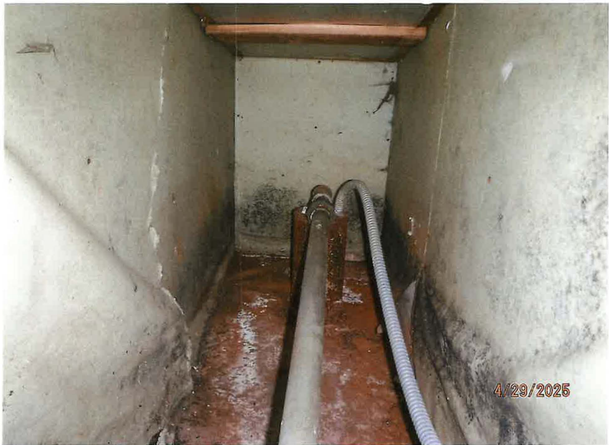
POD – GROUND WATER CASSED WELL 96-91-N-154
