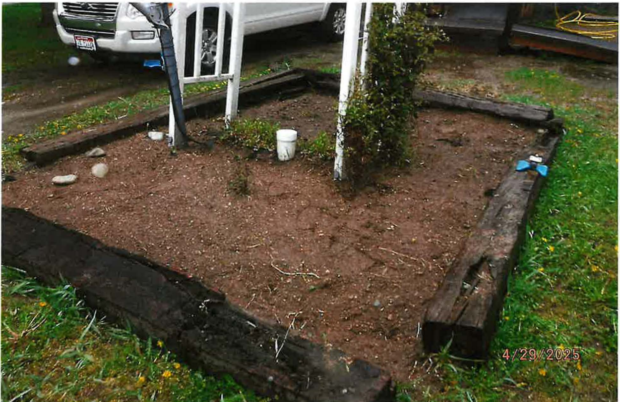
WATER CONVEYANCE SYSTEM – 9 EA WATER SERVICE LATERAL LINES OFF MAIN SERVICE PIPELINE (WHITE PVC RISER WITH CAP)
