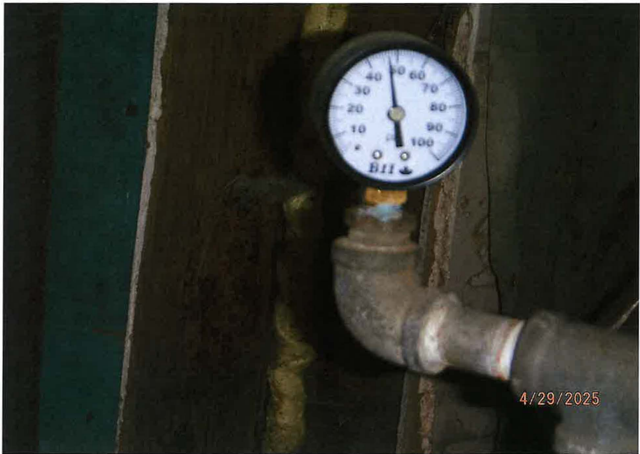
WATER SYSTEM PRESSURE MAINTAINS 45 PSI
