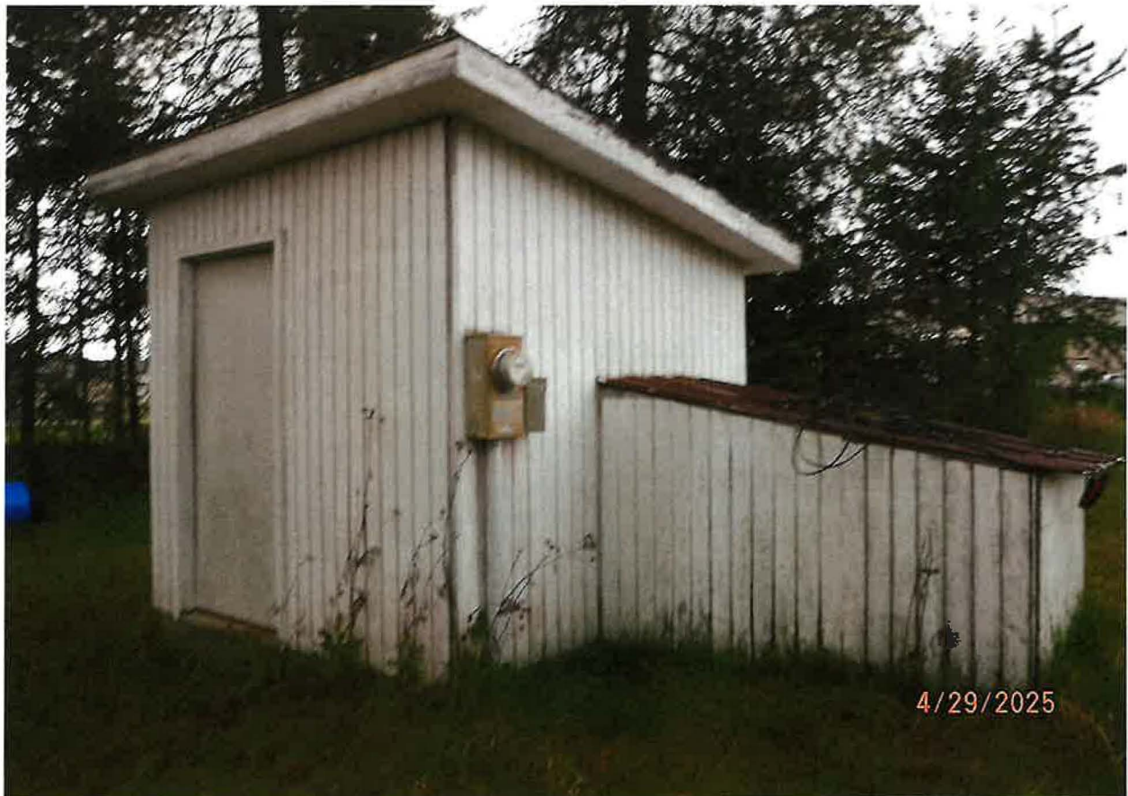
POD – GW WELL (SMALL DOG HOUSE TO RIGHT) AND PUMP STATION (LEFT HAND STRUCTURE)
