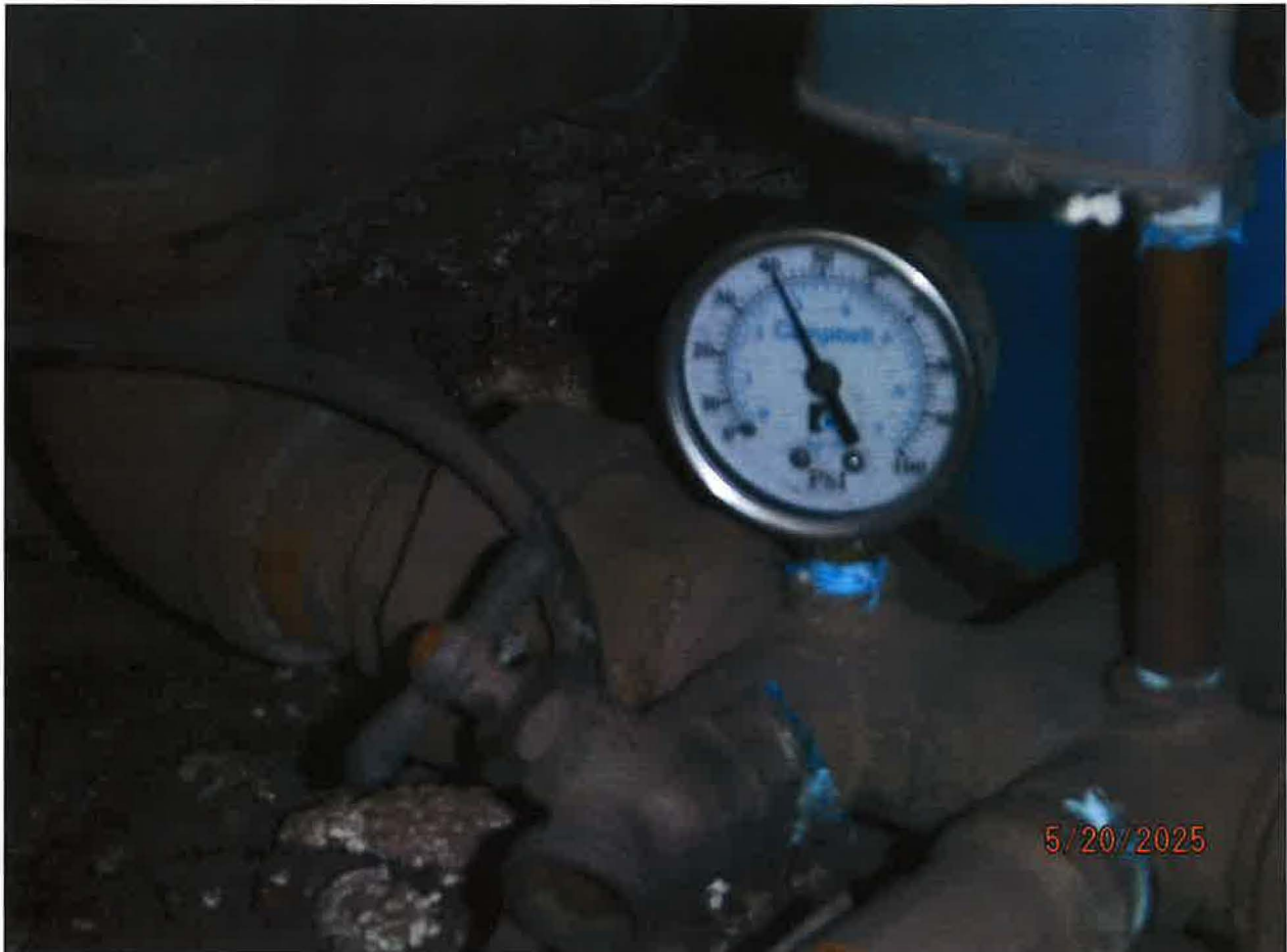
WATER CONVEYANCE SYSTEM – 2EA PRESSURE TANKS LOCATED WITHIN PUMP STATION WITH SYSTEM PRESSURE HOLDING AT 40-45 PSI
