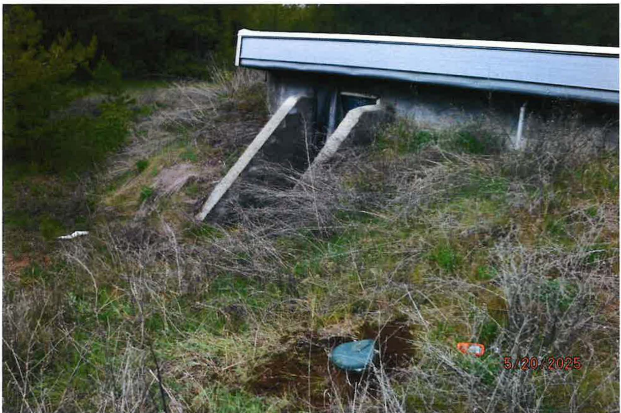
POD – GROUND WATER WELL, 6-INCH CASED WELL CO-LOCATED WITH PUMP STATION
