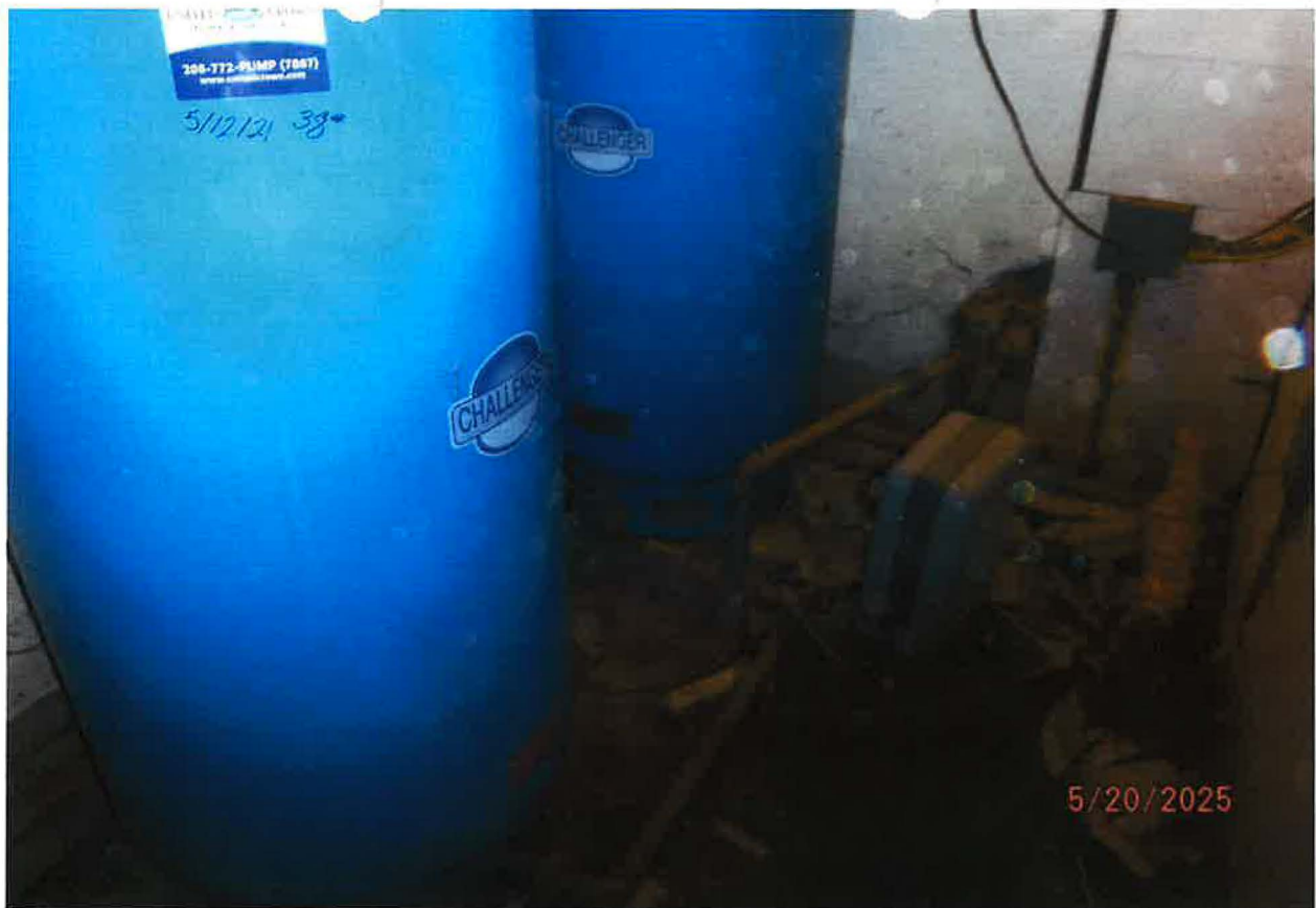
WATER CONVEYANCE SYSTEM – 2EA PRESSURE TANKS LOCATED WITHIN PUMP STATION WITH SYSTEM PRESSURE HOLDING AT 40-45 PSI
