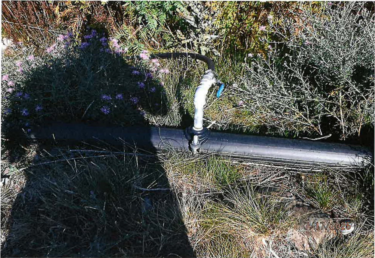
INDUSTRIAL / FIRE PROTECTION POU – 6 INCH PIPELINE WITH EXAMPLE OF 1-INCH RISER PIPELINE TO LOG DECK WATERING WITH IMPACT SPRINKLER(S)
