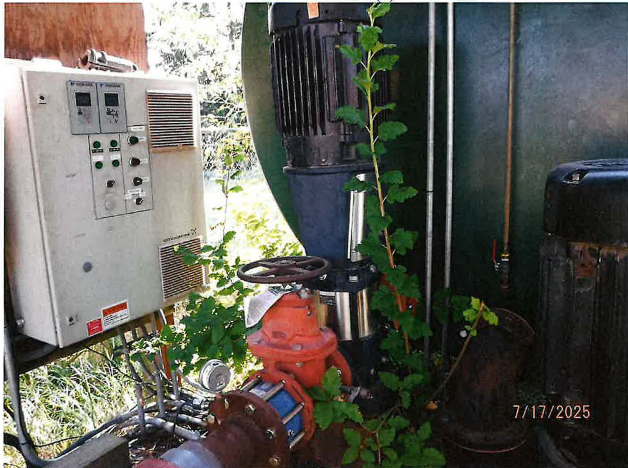
EXAMPLE – 1-OF-3 BALDOR MOTOR 25 HP TRANSFER PUMPS USED TO DISTRIBUTE WATER FROM RESERVOIR TO POU FOR INDUSTRIAL/FIRE PROTECTION USE(S)
