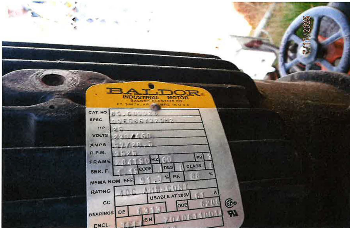
EXAMPLE – 1-OF-3 BALDOR MOTOR 25 HP TRANSFER PUMPS USED TO DISTRIBUTE WATER FROM RESERVOIR TO POU FOR INDUSTRIAL/FIRE PROTECTION USE(S)
