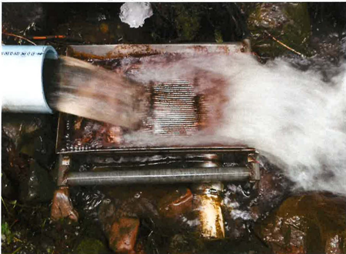
POD – 4-INCH PIPE IN CREEK ROUTES TO PENSTOCK THROUGH A SCREENED INFLOW COLLECTION PLATE
