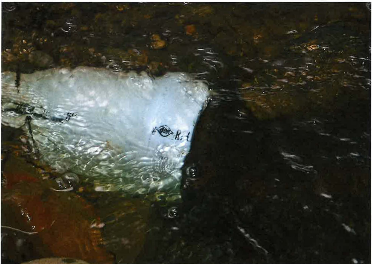
POD – 4-INCH PIPELINE PENSTOCK IN CREEK GRAVITY FLOWS WITH 181 FT OF HEAD
