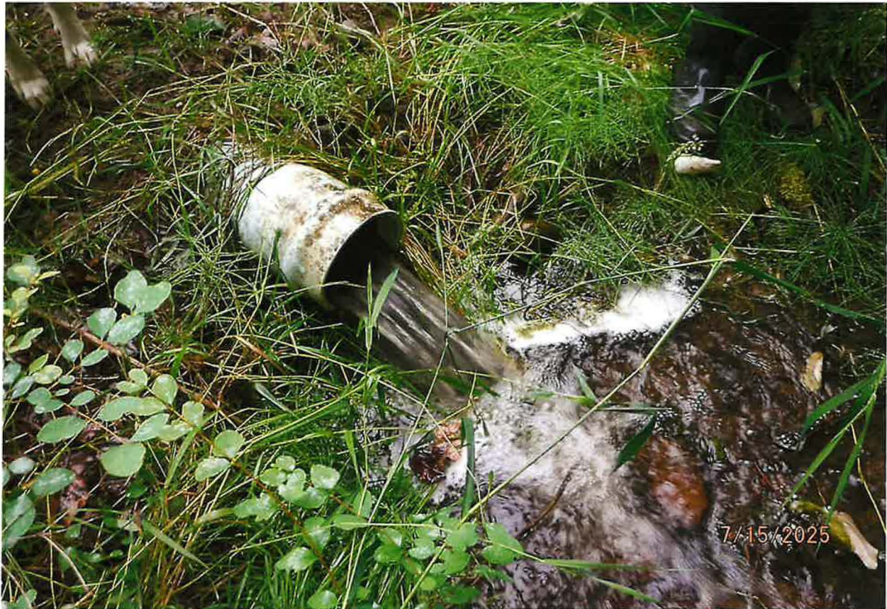
POU – POWER SYSTEM OVERFLOW DISCHARGE THROUGH 4EA 1/4-INCH NOZZLES AND MICRO HYDRO UNIT RETURN TO UNNAMED STREAM (NON-CONSUMPTIVE USE)
