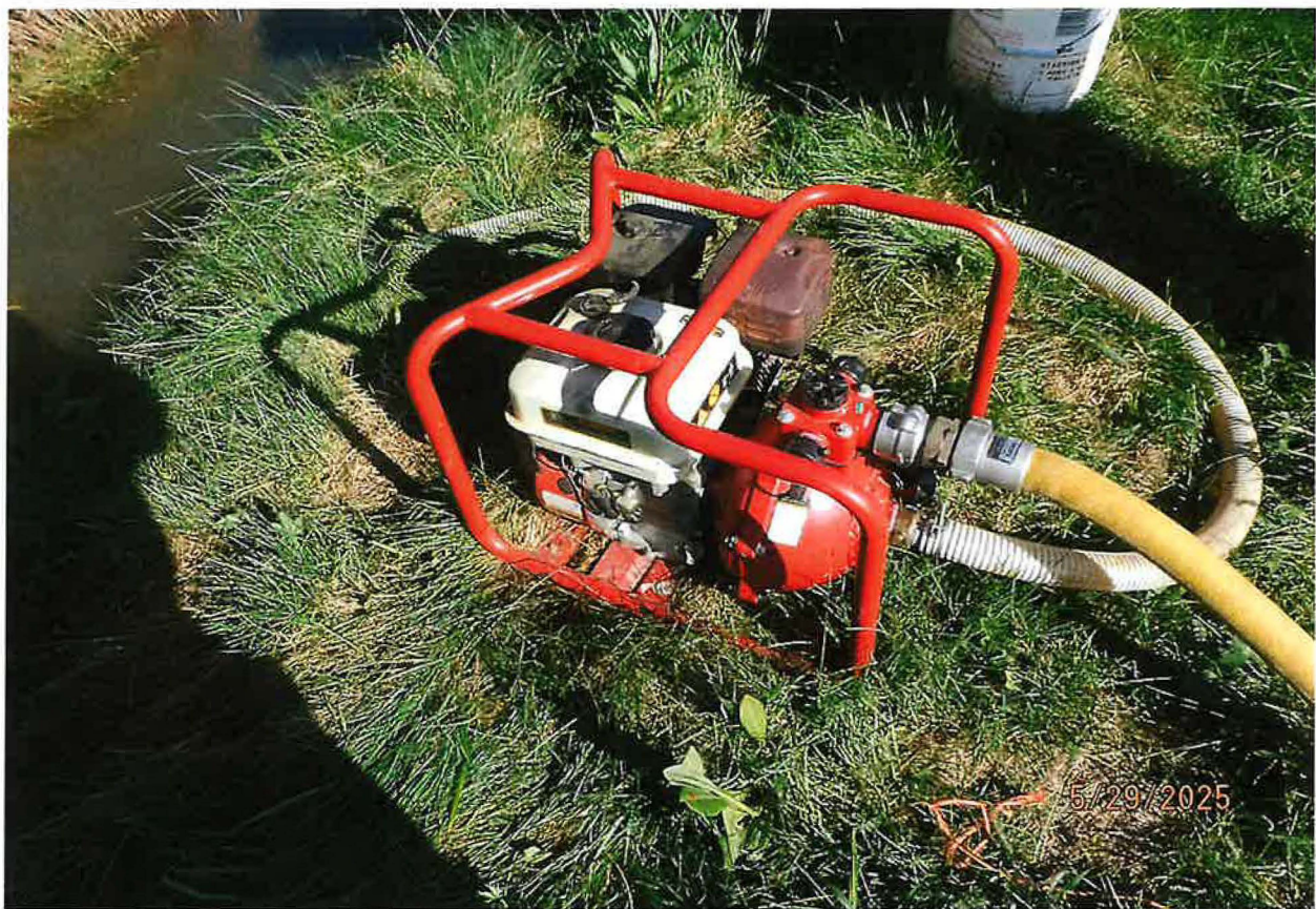
POD – DIVERTING WORKS USES A GENERATOR FRAMED WATER TRANSFER PUMP
