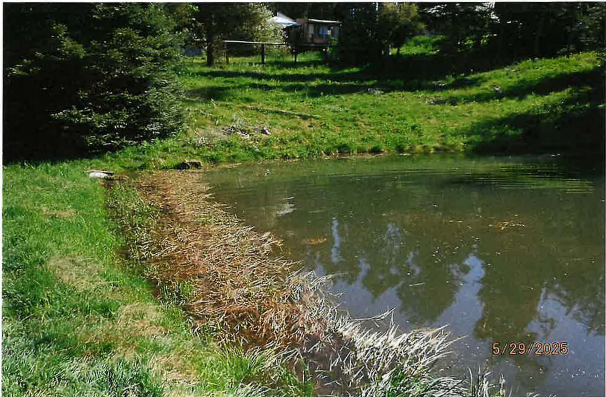
POD – EARTHEN DAM IMPOUNDS SURFACE RUNOFF SOURCE WATER AND SPRING SOURCE WATER IN THE STORAGE POND. THE POND WAS EXCAVATED WITH THE SPRING SOURCE BEING WITHIN THE HIGH WATER MARK OF THE POND
