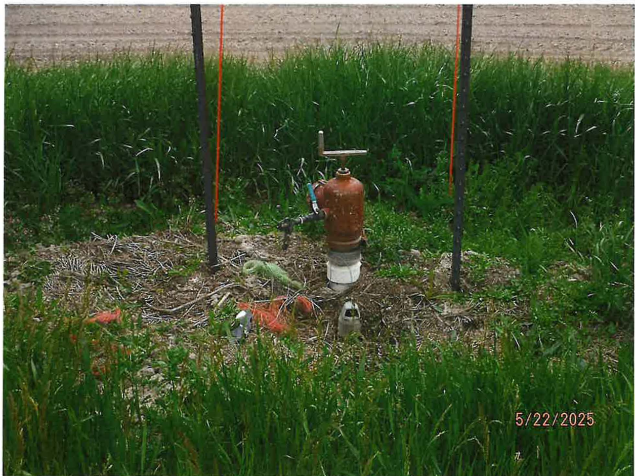
TWO (2) IRRIGATION RISER POINTS ON EASTERN SIDE OF DRAINAGE DITCH USED TO IRRIGATE WITH HAND LINE SPRINKLERS
