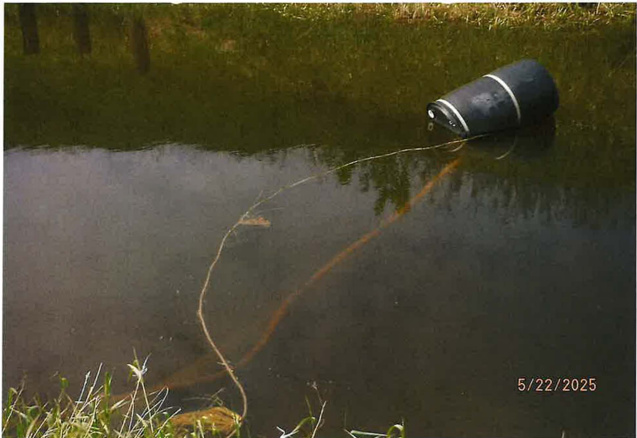
DIVERTING WORKS – FLEXIBLE 6-INCH INTAKE HOSE WITH SCREEN ATTACHED TO CORNELL CENTRIFUGAL PUMP SUCTION FLANGE
