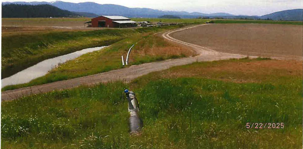
IRRIGATION WATER CONVEYANCE SYSTEM – APPROXIMATELY 1,000 FT OF 8-INCH ROUTES FROM POD, UP OVER/THROUGH DIKE EMBANKMENT, TO DISTRIBUTE WATER TO A CENTER PIVOT, A LATERAL WHEELED ‘MARCHING’ PIVOT, AND 2EA LATERAL HAND LINE IRRIGATION RISERS.
