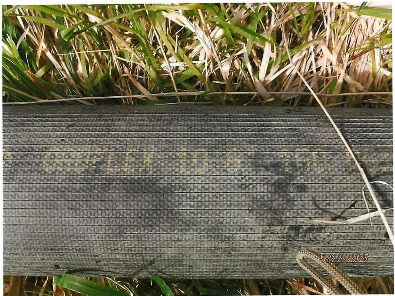
POD – CORNELL PUMP HAS A 3-INCH DISCHARGE ORIFICE THAT IS COUPLED UP TO A 6-INCH SOLID FLEXIBLE RUBBER HOSE
