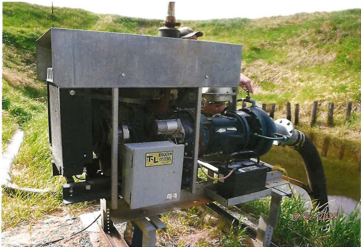
POD – DIVERTING WORKS INCORPORATE A CORNELL BRAND CENTRIFUGAL PUMP MODEL NO. 3RB-EM16, DIESEL FUEL POWERED PUMP
