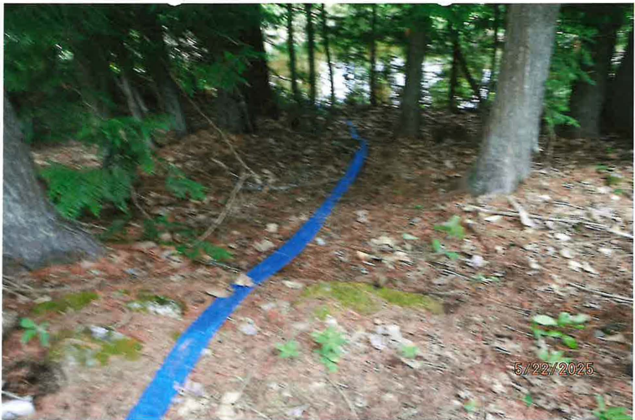
IRRIGATION FROM STORAGE – WATER PUMPED VIA 1.5-INCH FLEXIBLE FIRE HOSES (MULTIPLE) TO FILL TEMPORARY STORAGE TANK(S)
