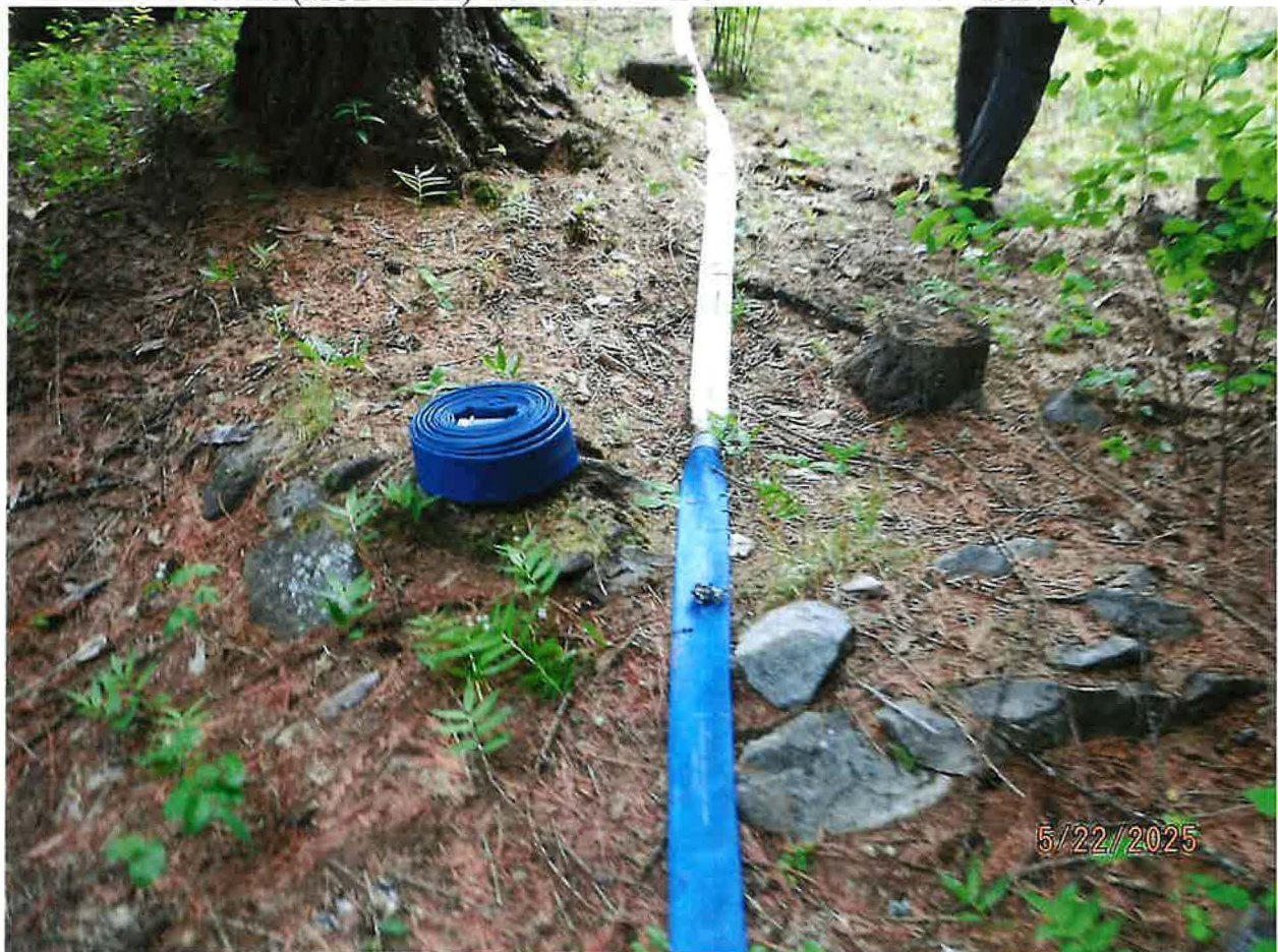
IRRIGATION FROM STORAGE – WATER PUMPED VIA 1.5-INCH FLEXIBLE FIRE HOSES (MULTIPLE) TO FILL TEMPORARY STORAGE TANK(S)
