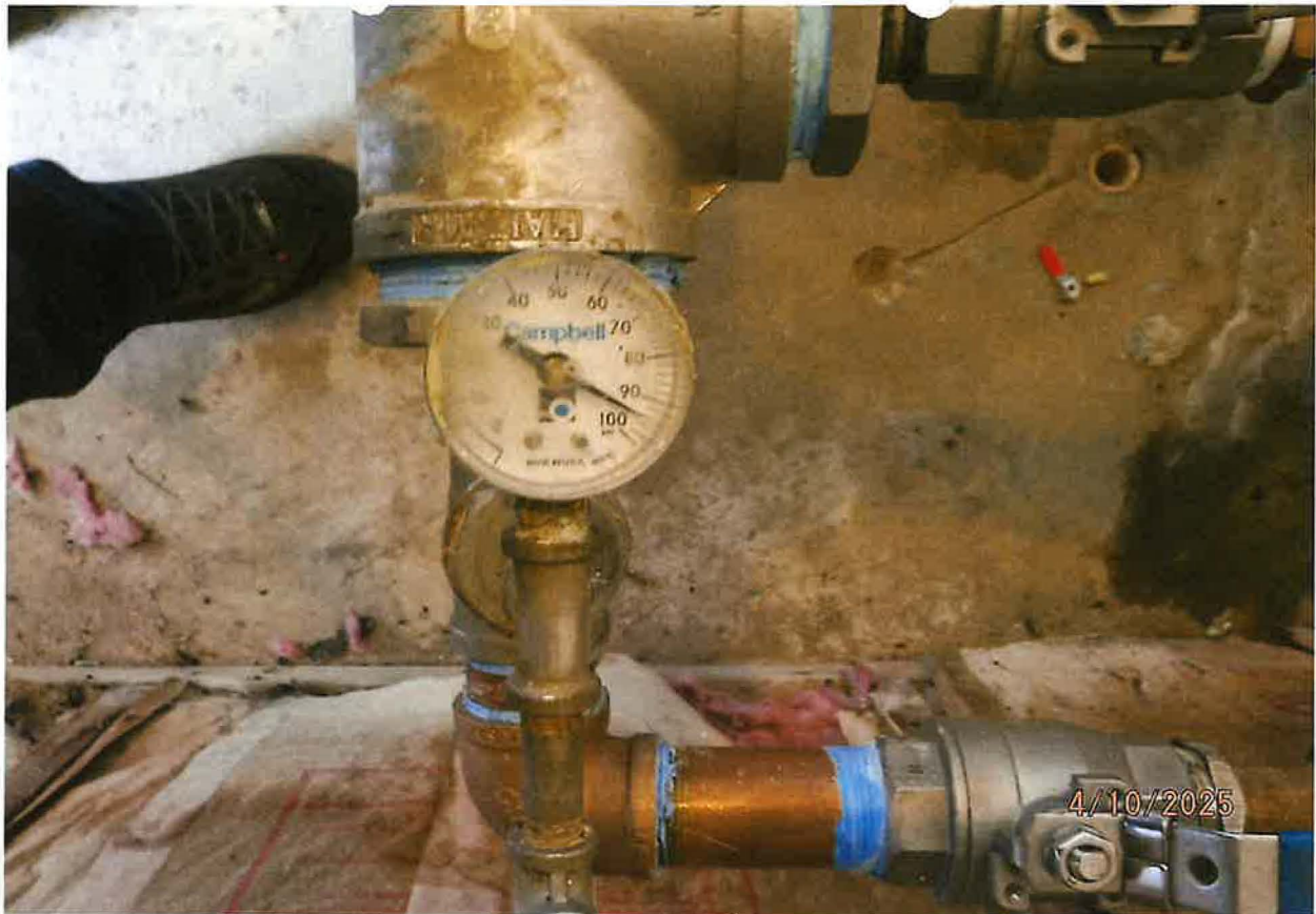
WATER SYSTEM 95 PSI OPERATING PRESSURE
