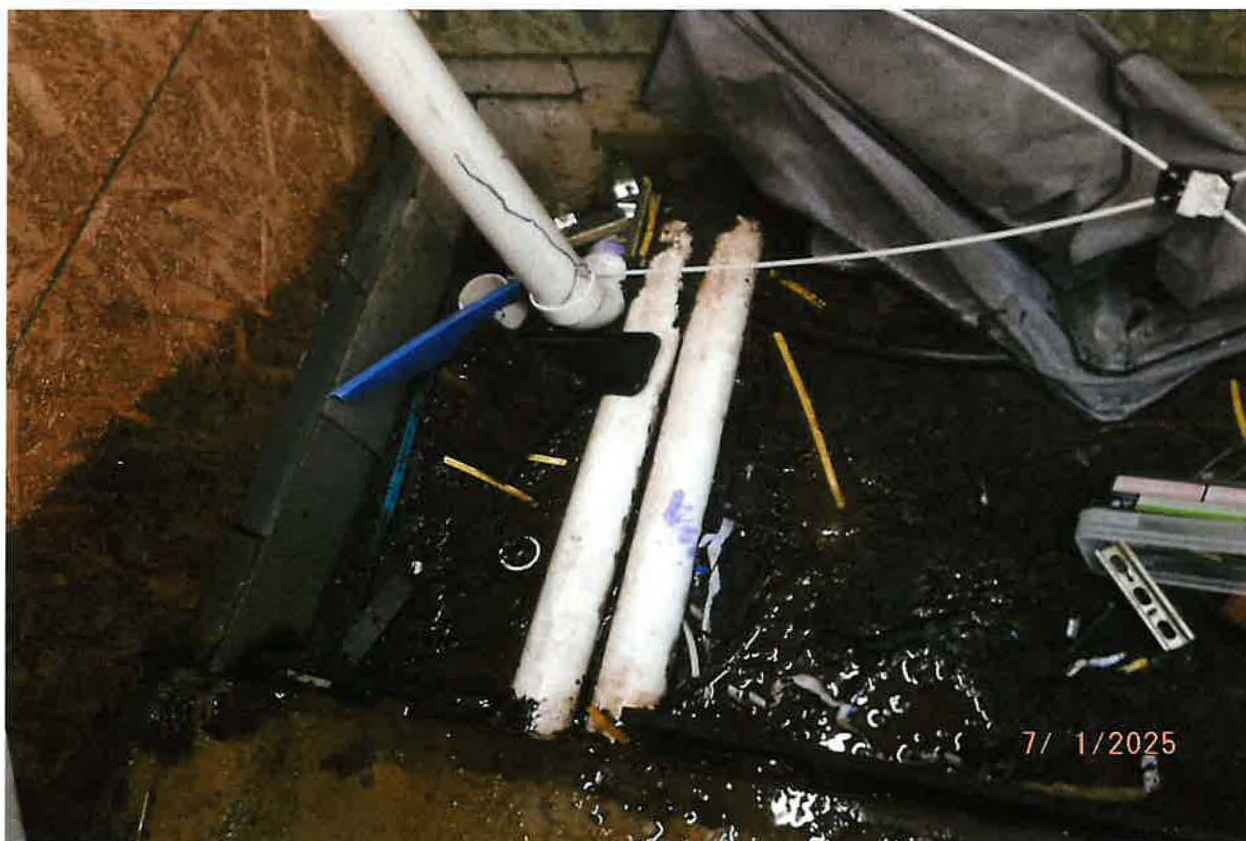
OVERFLOW DISCHARGE PIPES (2EA) IN ORDER TO CAPTURE ALL WATER THROUGH NOZZLES WITHOUT FILLING UP BLUE COLLECTION BIN
