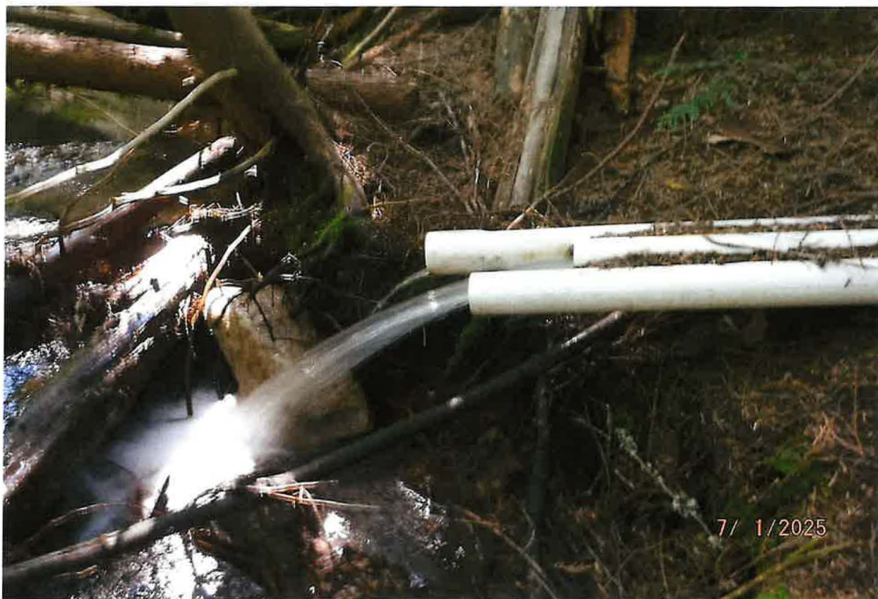
POWER POU – OVERFLOW DISCHARGE RETURNED DIRECTLY TO FLUME CREEK (NON-CONSUMPTIVE USE)
