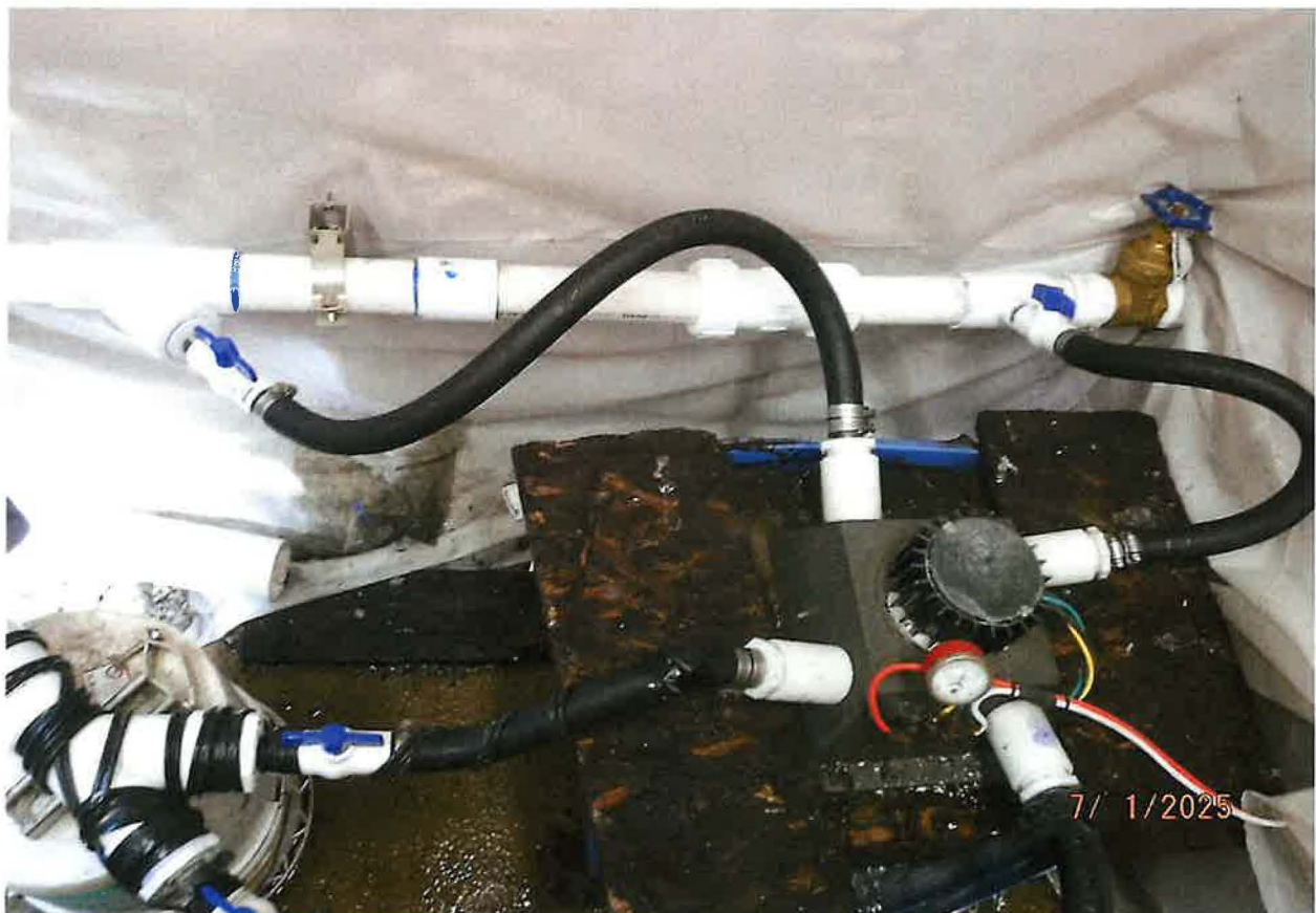
POWER POU – PELTON WHEEL MICRO HYDRO WITH FOUR (4) ACTIVE NOZZLES IN POWER PRODUCTION
