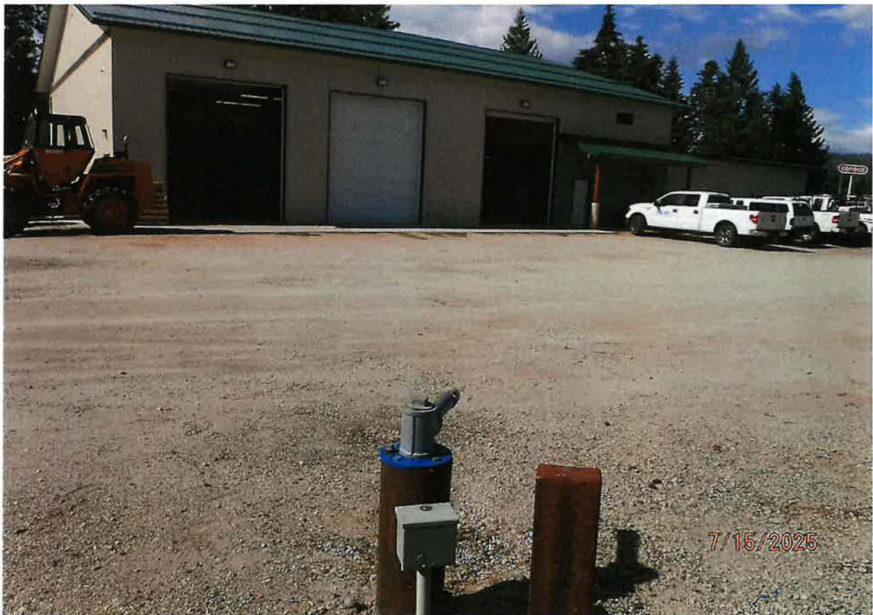
POD - 8-INCH CASED GROUND WATER WELL
