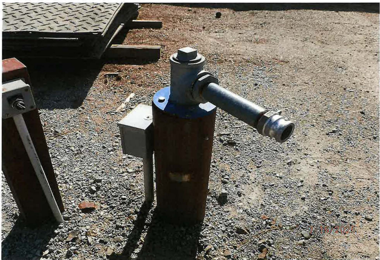
INDUSTRIAL POU – WELL CAPPED WITH WATER TRUCK FILL POINT ADAPTER – INDUSTRIAL USE TO FILL WATER TANKS/TENDER TRUCKS IN SUPPORT OF WELL CONSTRUCTION ACTIVITIES.
