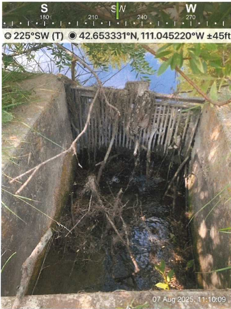
The screen at the diversion inlet from a side channel of Crow Creek. Beaver activity explains the condition of the screen.
