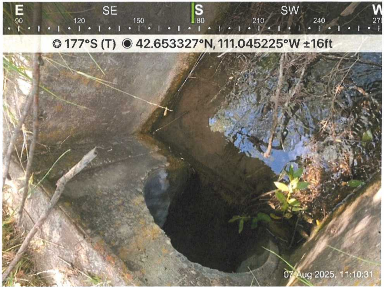
The entrance to the underground pipe at the diversion.
