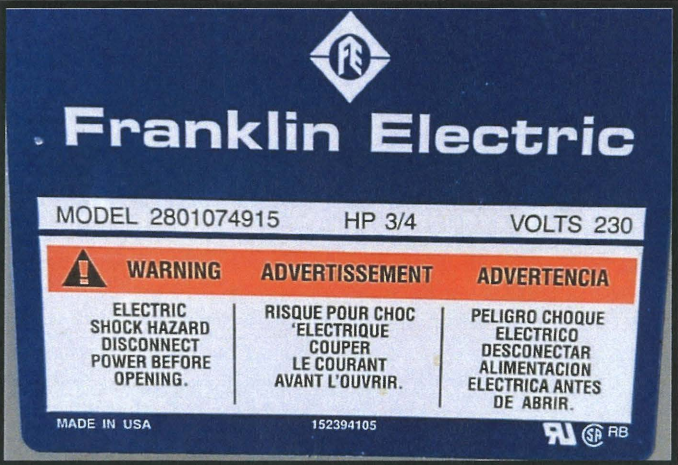
Photo 26- Submersible pump spec label for domestic/stockwater well.
