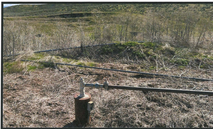
Photo 17- Cistern well #2 located north of the cistern. The main to cistern well #3 is in the background.
