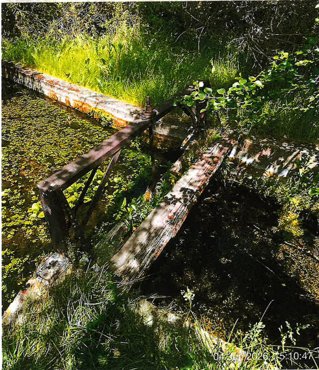
Partially open headgate at the point of diversion. Dimensions are 5ft wide x ~2ft deep. Headgate was only open an inch or two at the bottom.
