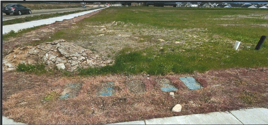
Photo 26- At the corner identified above, facing north. The 6" stub out valves are in the right of the image and the control valves for the future irrigation system are installed. However, the escort noted during the examination that there is no irrigation in this area yet.
