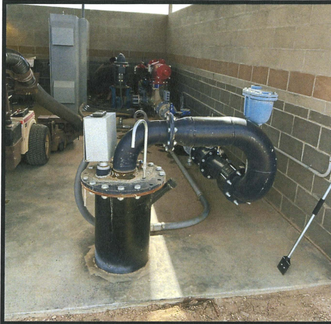
Photos 5 & 6- The ground water well in the foreground with the twin 30 Hp surface water pumps (red pumps) in the background with the surface water flowmeter to the right of them(right image), at the southeast corner of the pump house. A manual shutoff valve between the flow meters can be opened to allow the system to be charged by the well.
