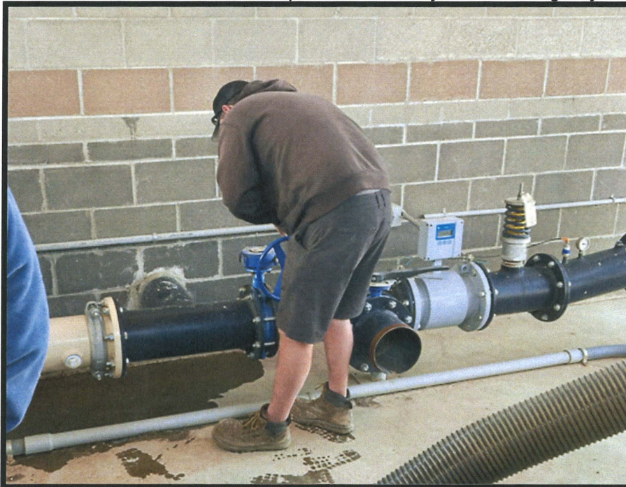
Photo 7- Escort opening the valve on the left of the groundwater flowmeter prior to charging the system for the field examination.
