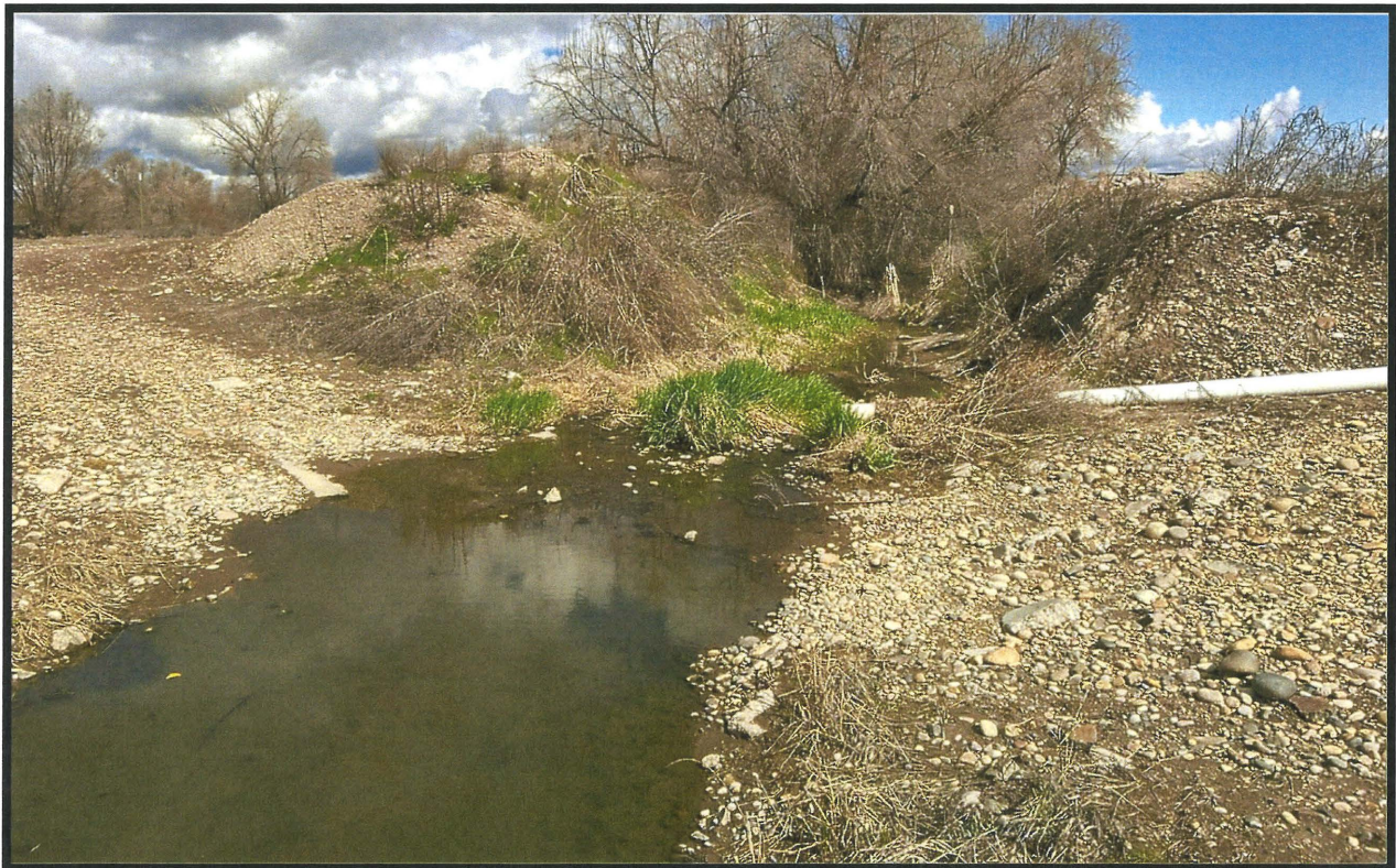
Photo 2-Facing north, downstream on the drainage. White pipes carry runoff from the adjacent fields into the drainage when irrigation takes place later in the season.
