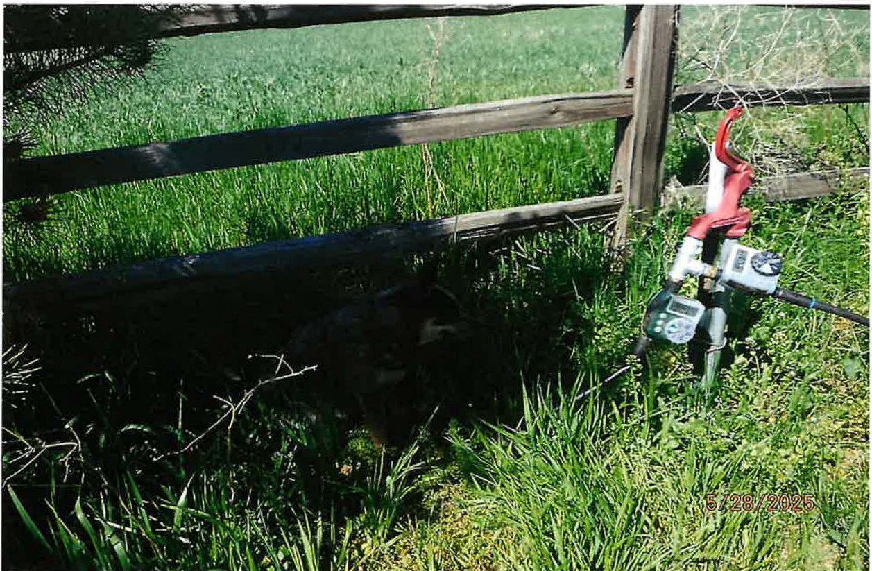
IRRIGATION POU – NORTHWEST MOST HYDRANT AND SOAKER HOSE ZONE THAT IRRIGATES ALONG WIND ROW FENCELINE
