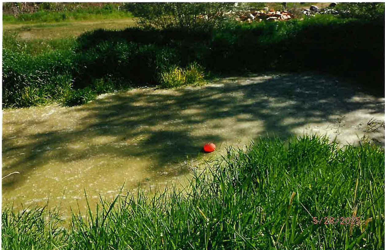
ORANGE BALL INDICATES LOCATION OF FOOT VALVE INTAKE PIPE IN POOL
