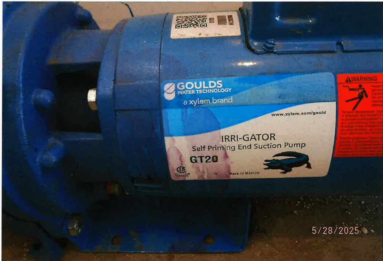
GOULDS GT20 SELF PRIMING PUMP END (2 HP)
