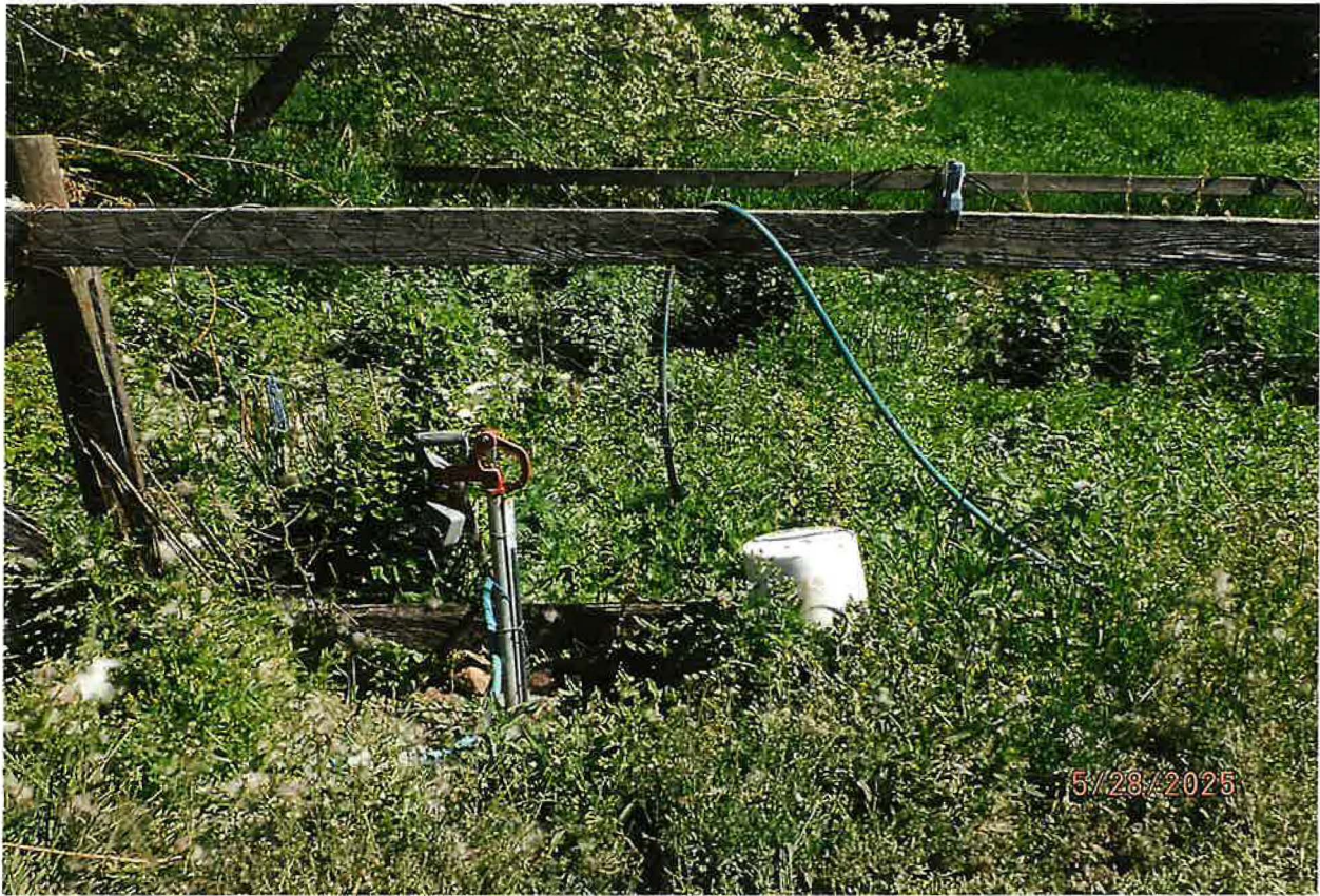
IRRIGATION POU - MULTIPLE GARDEN PLOTS WATERED USING FROST-FREE HYDRANT-TO-DRIP LINES AND HOSE WITH SPRAY NOZZLE
