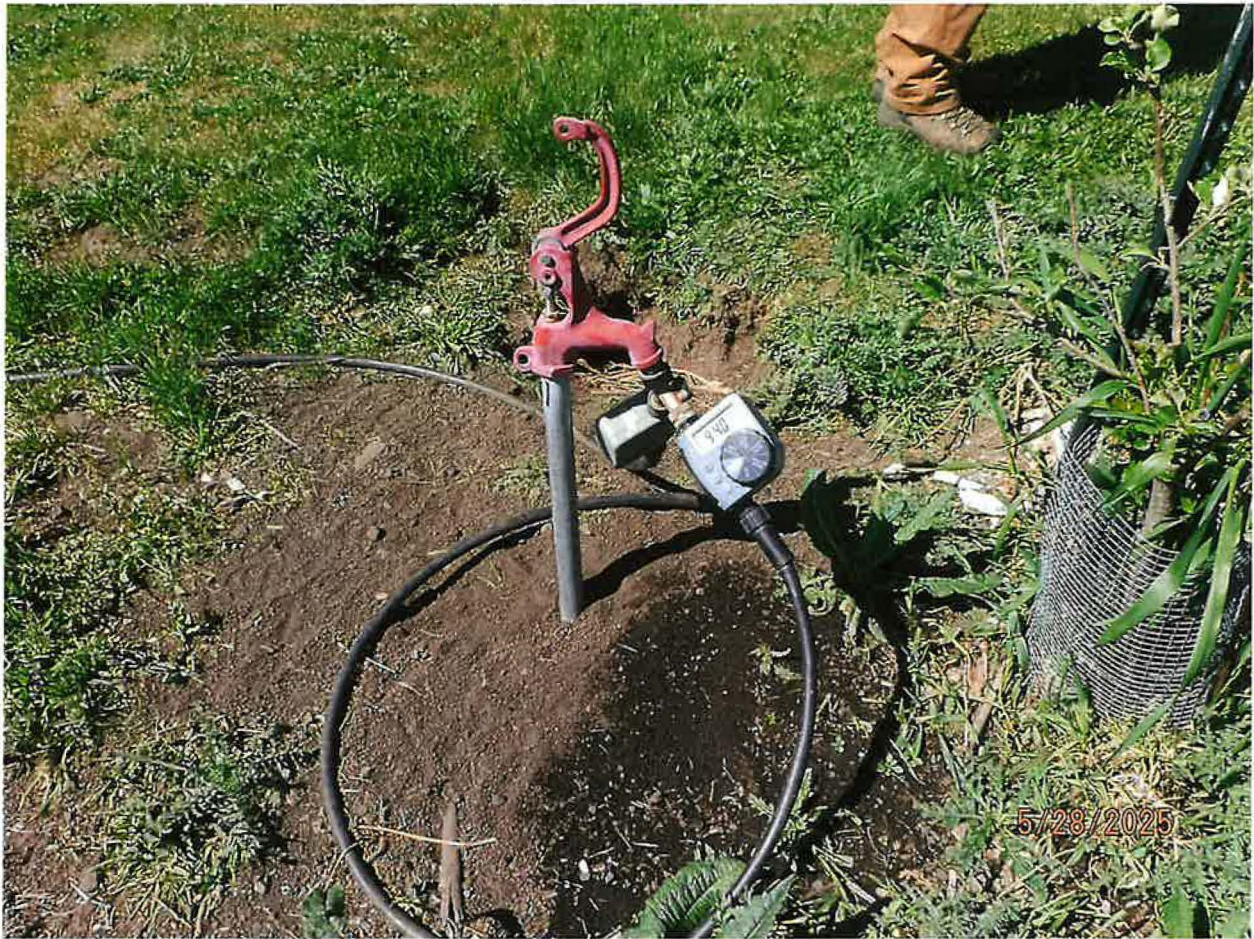
EXAMPLE – ONE OUT OF NUMEROUS (TO MANY TO COUNT) HYDRANTS AND TIMER OPERATED SPRINKLER ZONES
