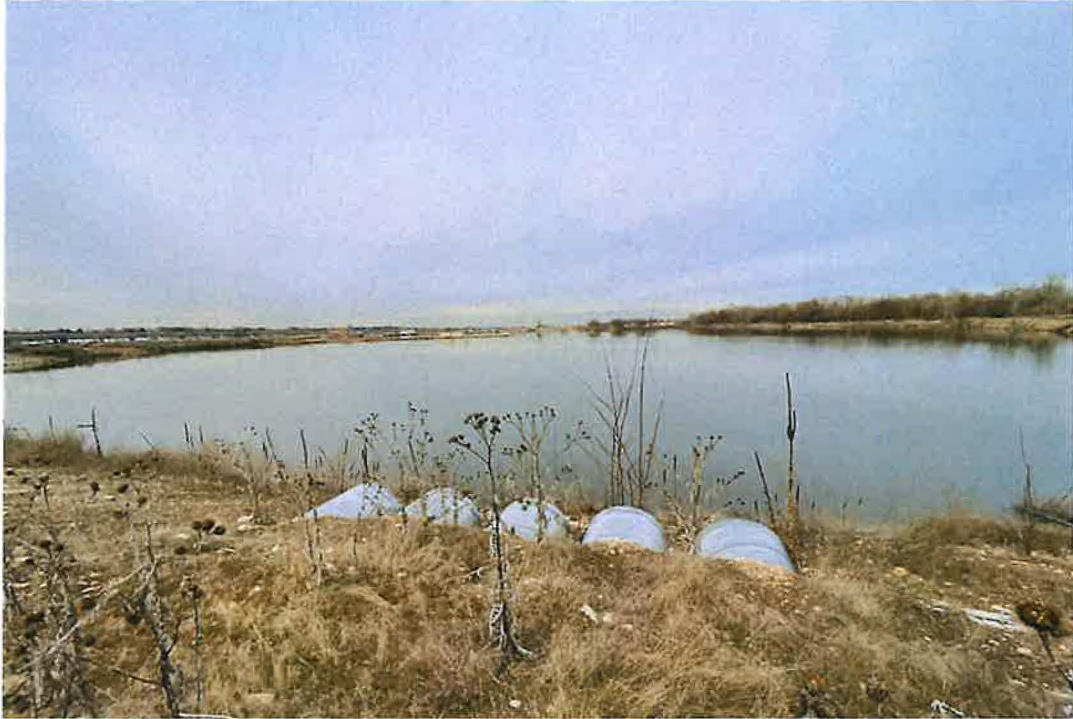
Figure 4 3" diameter pipes as part of the pit capture prevention system. These pipes are located on the Northeast end of the pond and are featured in the system diagram in figure 1.
