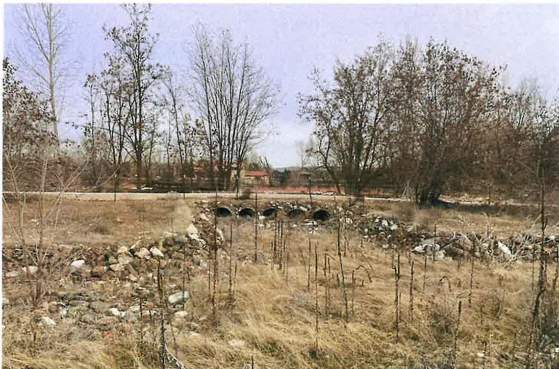
Figure 7 Photo facing North, taken at North end of the pond. The photo features five 3' diameter pipes that provide prevention for pit capture.
