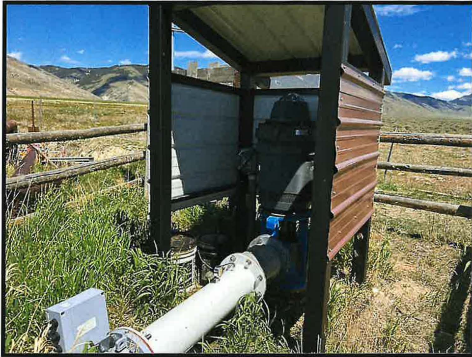
Photo 1- Irrigation well head and pump, adjacent to abandoned surface water source POD.
