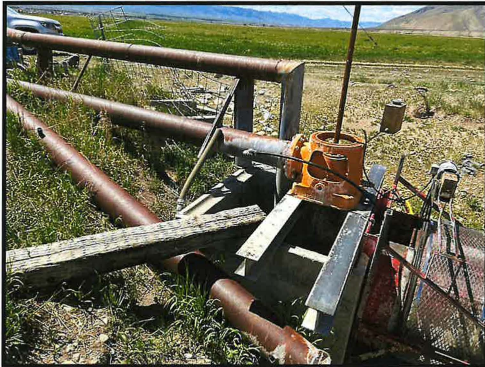
Photo 2- Facing west- Abandoned surface water diversion screen adjacent to irrigation wellhead. New POD is to the southeast.
