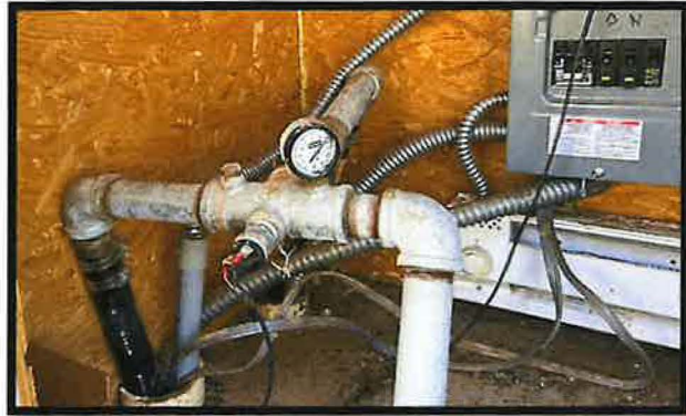
Photo 7-(Left) Pump controller with evident damage. Photo 8-(Right) 2" Poly line from pump to Manifold with broken pressure gauge. 1 1/2" Poly line goes out through chase in the corner.
