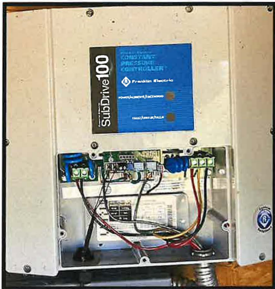
Photo 7-(Left) Pump controller with evident damage. Photo 8-(Right) 2" Poly line from pump to Manifold with broken pressure gauge. 1 1/2" Poly line goes out through chase in the corner.
