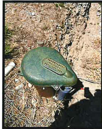
Photo 3-(Left) Pump house with well head visible next to a frost free spigot in the left of the image. Photo 4-(Right) Well head.
