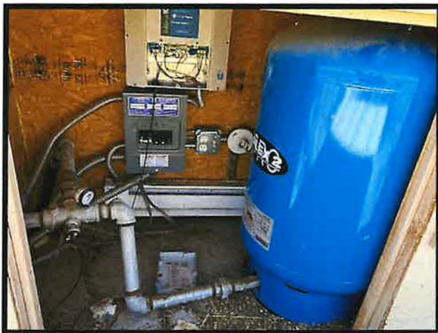
Photo 5 & 6- Pump VFD with parts and cover on the floor of the pumphouse next to the blue 44-Gallon pressure tank.
