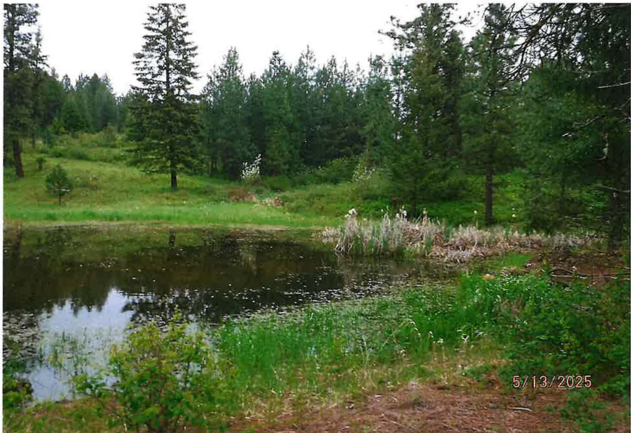
POD – ROAD CONSTRUCTED IN SMALL DRAINAGE SERVING AS EARTHEN DAM FOR STORAGE POND
