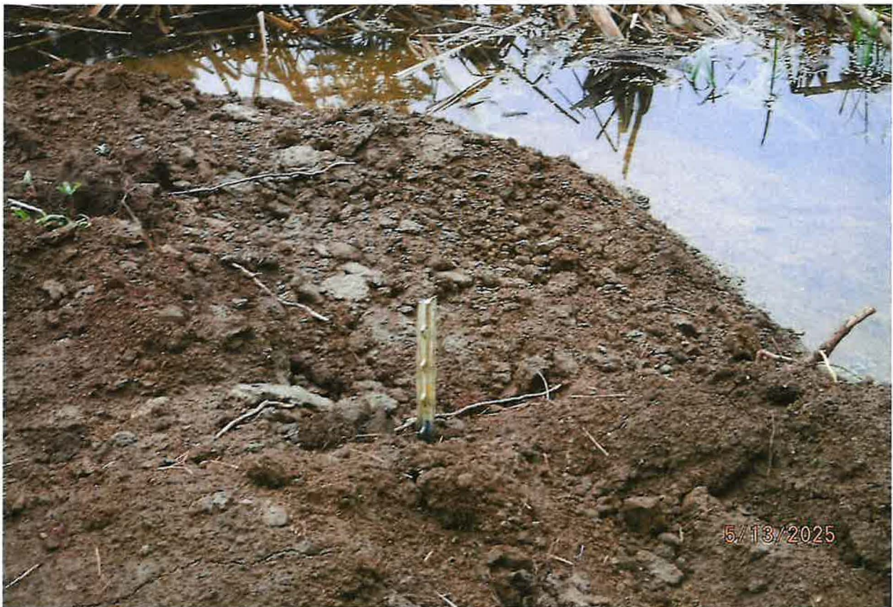
WHITE METAL FENCE POST DESIGNATES PROPERTY BOUNDARY (L/H) FILLED IN AND (R/H) MAINTAINED FOR STORAGE POND
