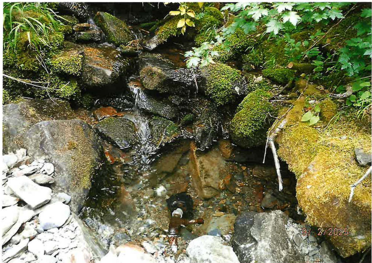
POD – 1-INCH SCREENED PENSTOCK PIPE IN UNNAMED STREAM
