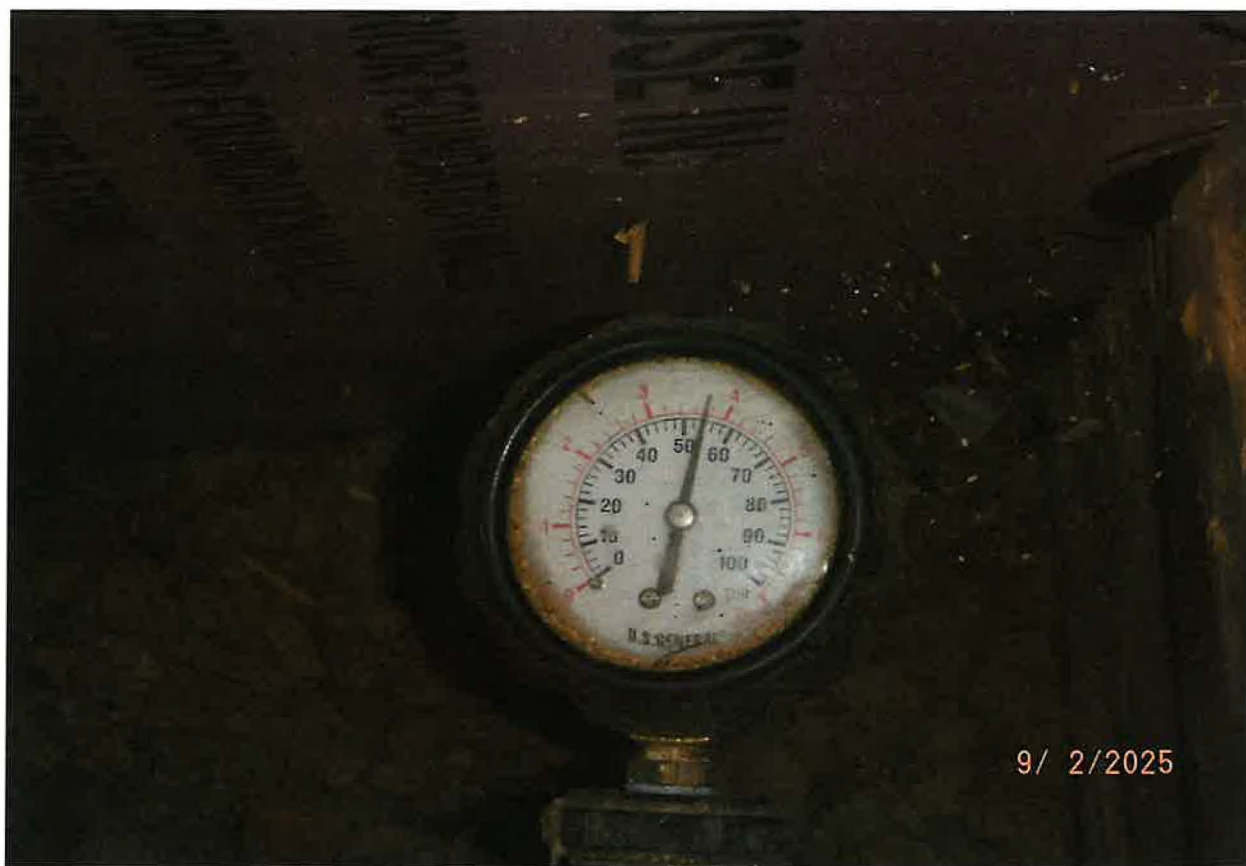
55 PSI OPERATING PRESSURE ON HYDRO POWER SYSTEM IN OPERATION
