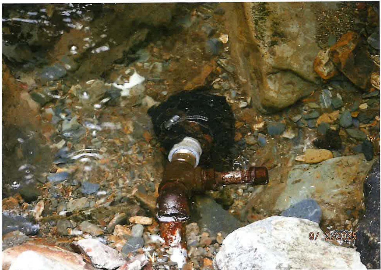
POD – PENSTOCK INTAKE PIPE ROTATES TO ALLOW PERIODIC CLEANING OF SCREEN
