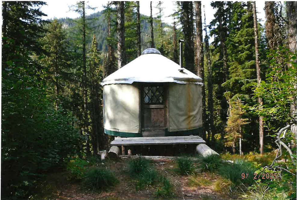
DOMESTIC POU – SMALL YURT RAISED ON PLATFORM; DEDICATED FROST-FREE HYDRANT PLUMBED TO CABIN FOR WATER USE BY HOSE
