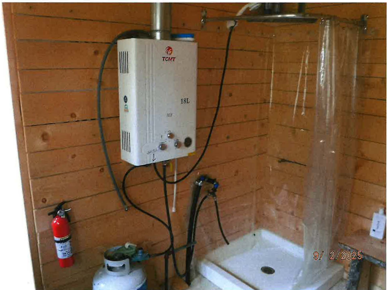
DOMESTIC POU – SMALL CABIN PLUMBED FOR BATH HOUSE (POWER UNIT LOCATED BENEATH RAISED CABIN)
