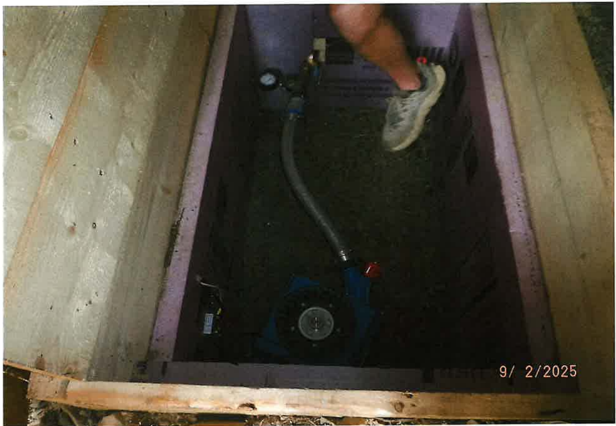
POWER POU – POWER STATION LOCATED BENEATH WOOD CABIN HAND DUG VAULTED CUBE
