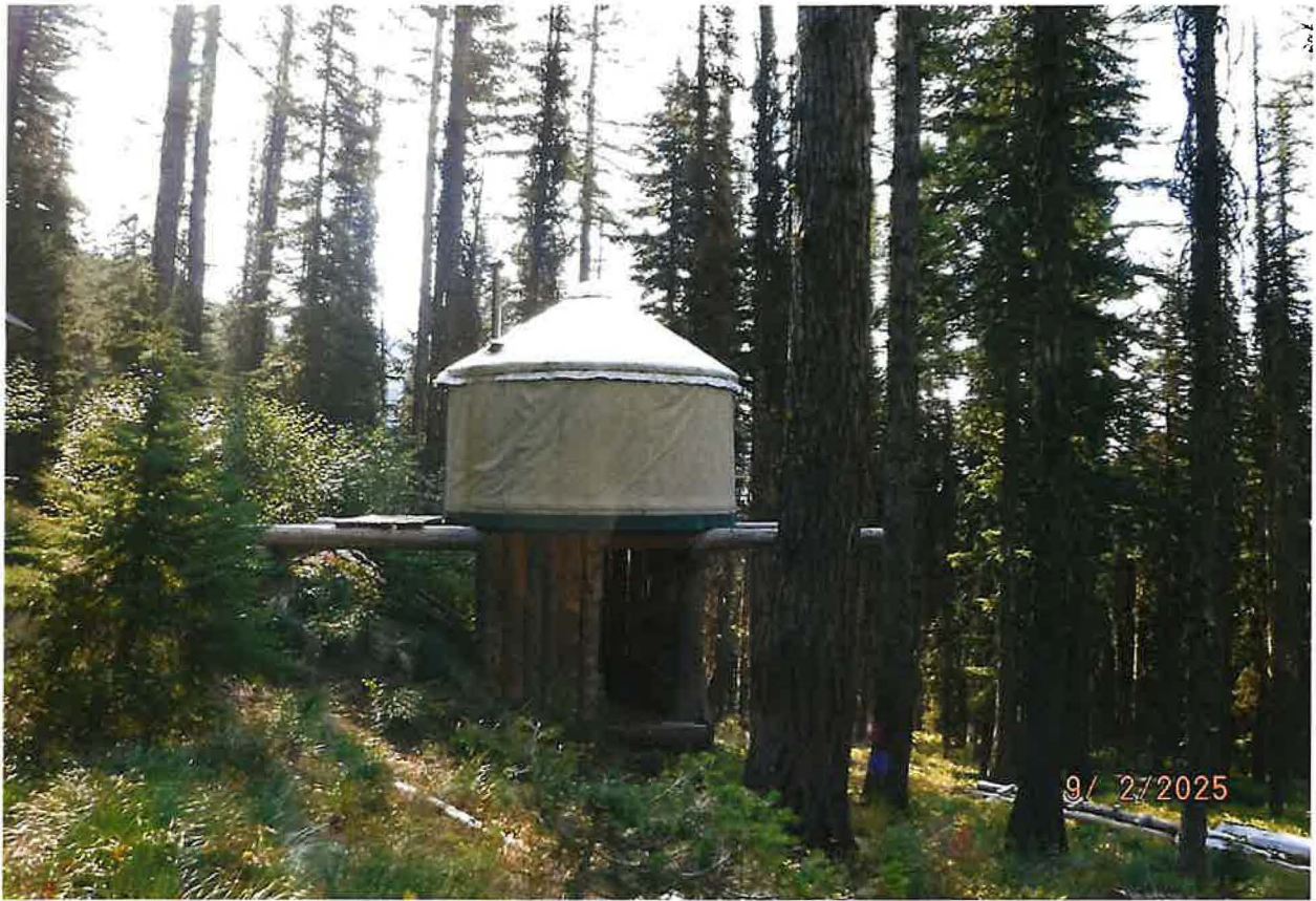
DOMESTIC – SMALL YURT; ALL THREE DOMESTIC STRUCTURES ARE ON RAISED STRUCTURES TO ACCOUNT FOR WINTERTIME SNOWPACK CONDITIONS
