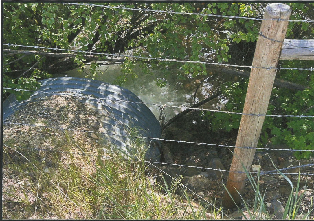
Photo 1- 2" Poly line exiting the north bank of Withington Creek and passing under the road through the culvert.
