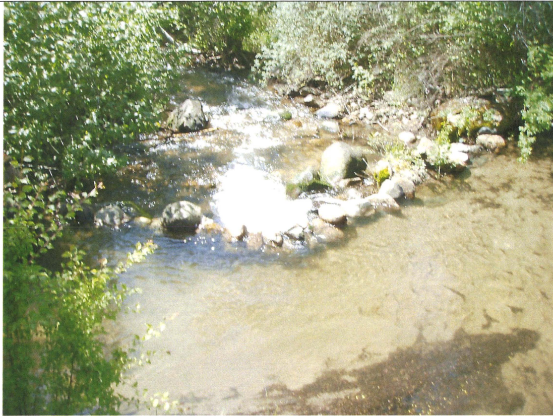
Figure 1. Diversion dam on Porter Creek.
