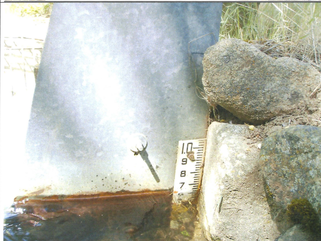
Figure 4. A staff gage on the side of the Cipolletti weir measure the depth of water over the crest of the weir.
