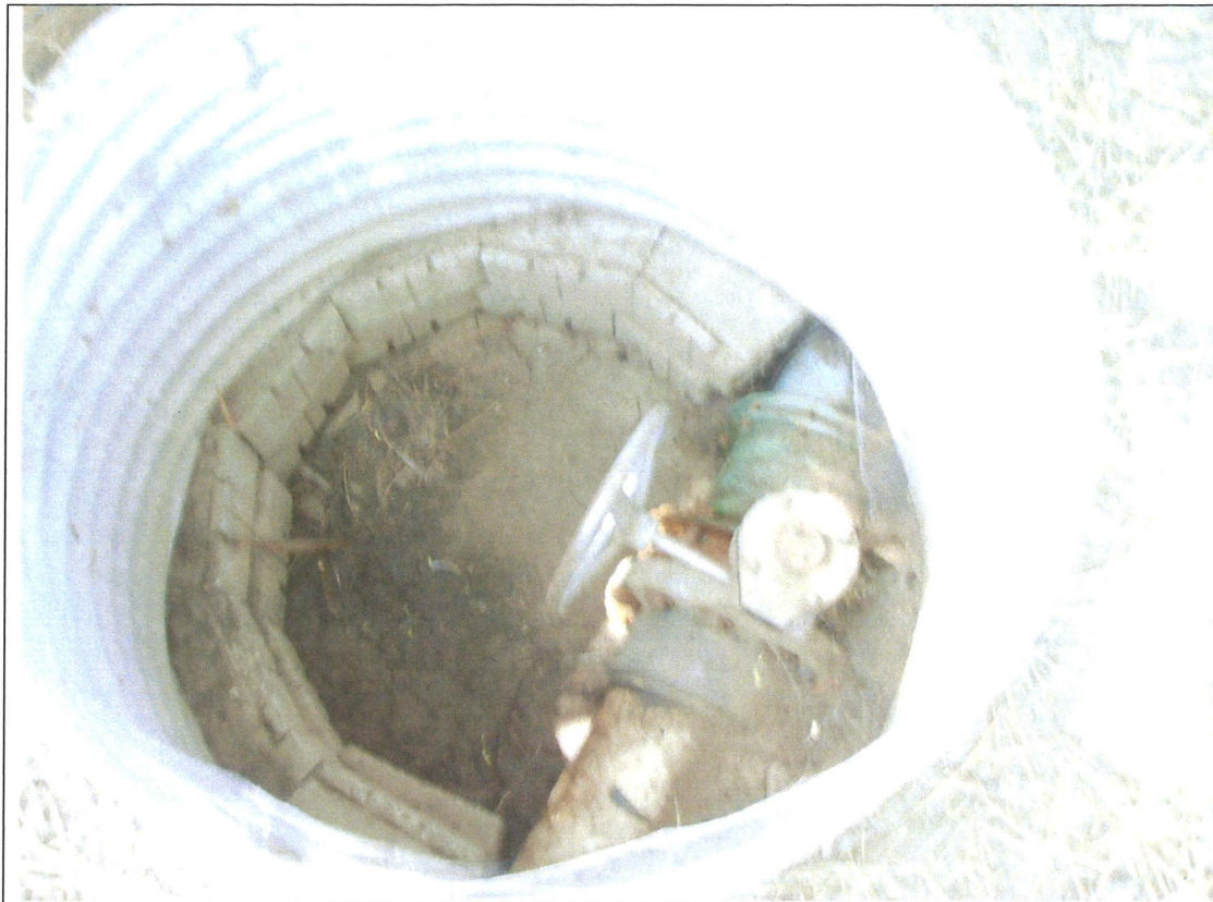
Figure 7. This shutoff valve located at 15 Maria Drive which is approximately 5,700 feet from the POD and turns off the entire mainline to Faull Ranch.
