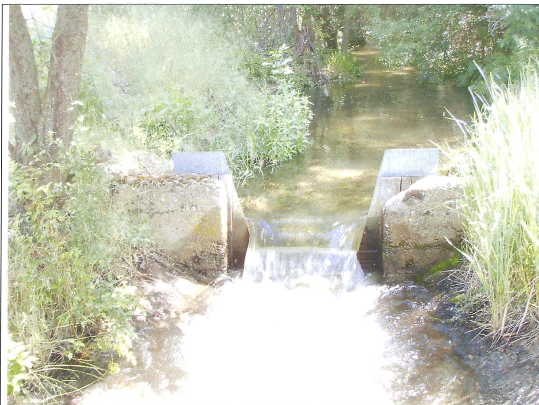
Figure 3. The Cipolletti or Trapezoidal Weir in the Faull Ranch diversion ditch has a 2.0 ft crest.
