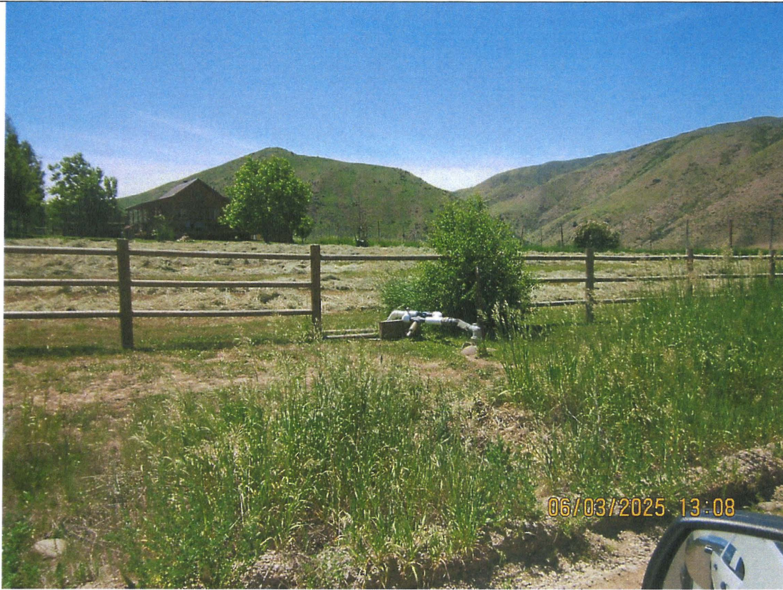
Figure 15. Stubb valve and irrigation at 22 Hill Creek Road.
