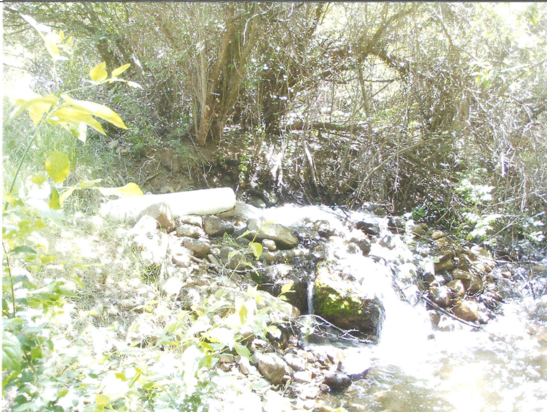
Figure 6. The outlet pipe for the bubbler carries any excess water immediately back to Porter Creek just upstream of the next Porter Creek Diversion for Woods/Bledsoe.
