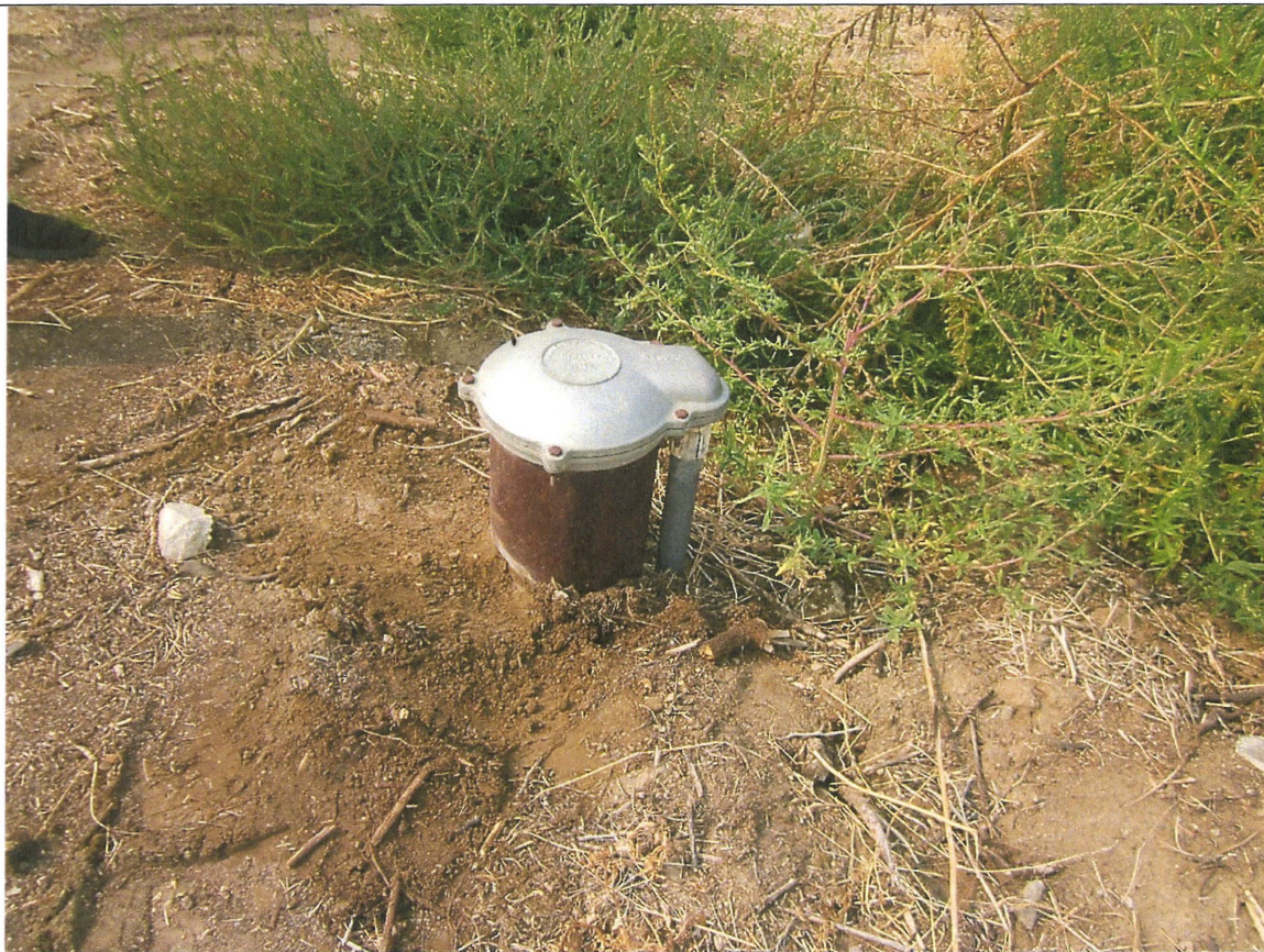
Figure 1. The source for the system is ground water from Well ID #304533, no metal tag.
