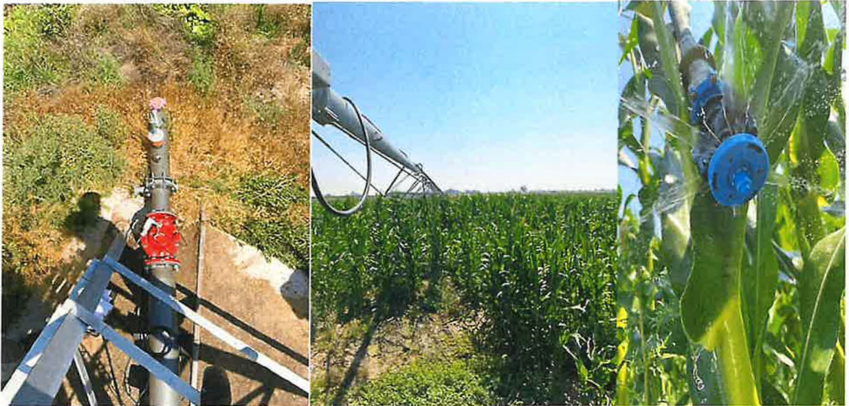
Photos 8-10, from left to right- (8)Pivot 1 looking down tower on control valve and pressure blow off. (9) Looking down the lateral line of pivot. (10) Nelson Sprinkler regulator with nelson rotator head (6 per span).
