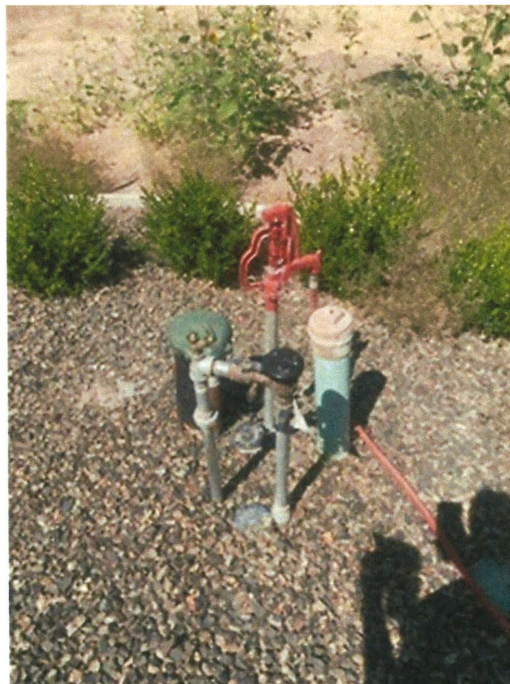
Figure 3 Photo of well head (point of diversion).
