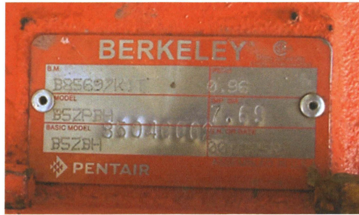
Figure 6 Motor specification tag displaying model number.
