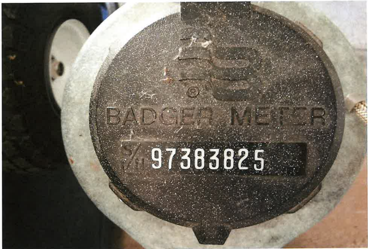
BADGER METER S/N 97383825 RECORDALL FLOWMETER INSTALLED PRIOR TO DISTRIBUTION TO STORAGE RESERVOIR
