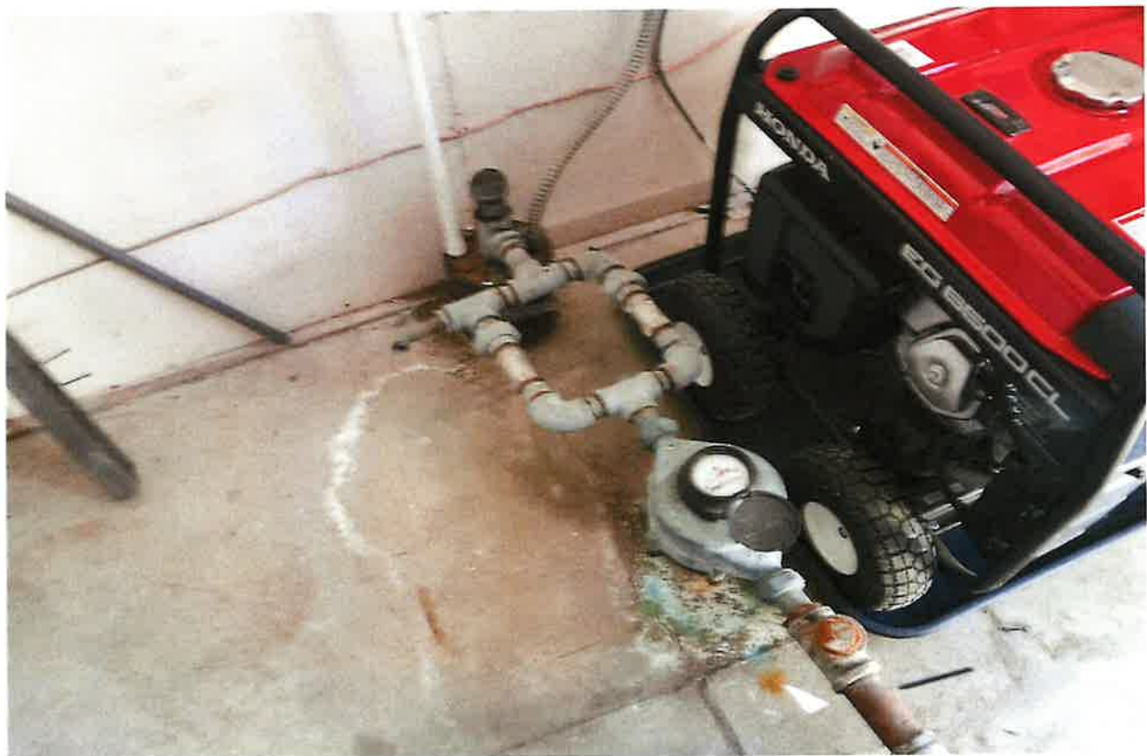
FLANGED VELOCITY STYLE FLOW METER INSTALLED AT WELL HEAD
