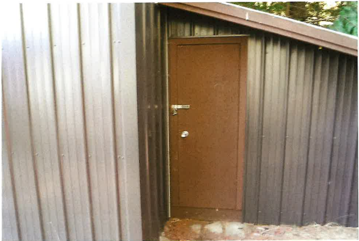
ENCLOSED STORAGE RESERVOIR STRUCTURE
