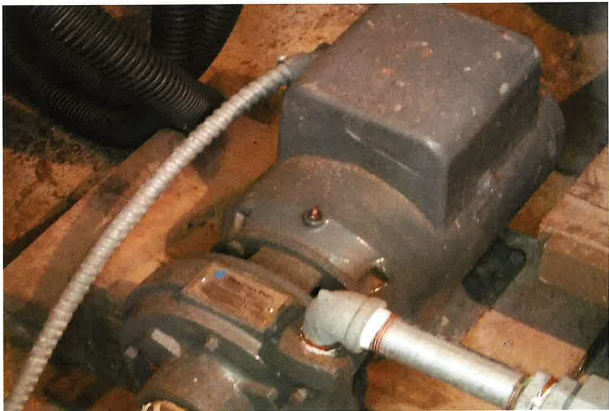
STORAGE RESERVOIR USES A CENTRIFUGAL DISTRIBUTION PUMP WITH PRESSURE TANKS TO DISTRIBUTE WATER TO DOMESTIC SYSTEM
