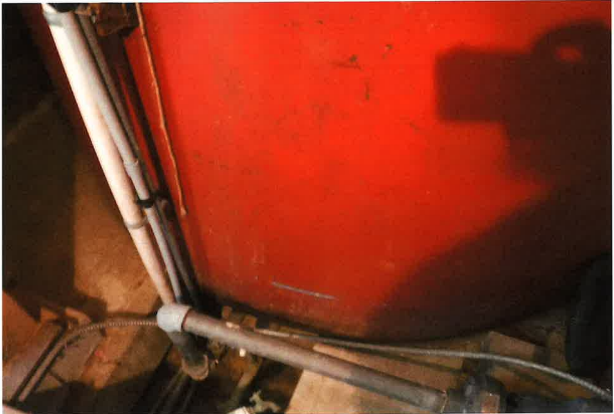
STORAGE RESERVOIR USES A CENTRIFUGAL DISTRIBUTION PUMP WITH PRESSURE TANKS TO DISTRIBUTE WATER TO DOMESTIC SYSTEM
