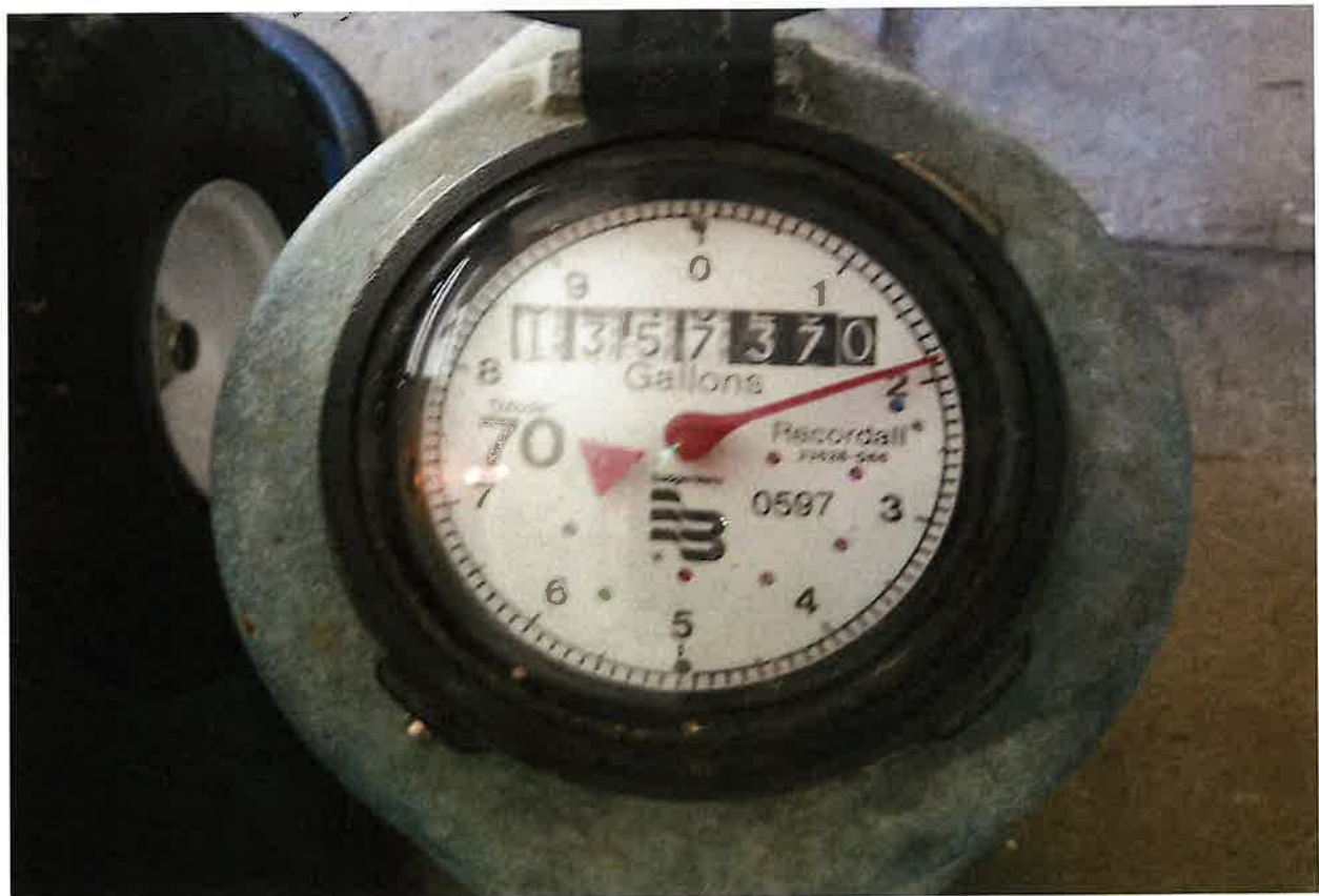
BADGER METER S/N 97383825 RECORDALL FLOWMETER INSTALLED PRIOR TO DISTRIBUTION TO STORAGE RESERVOIR
