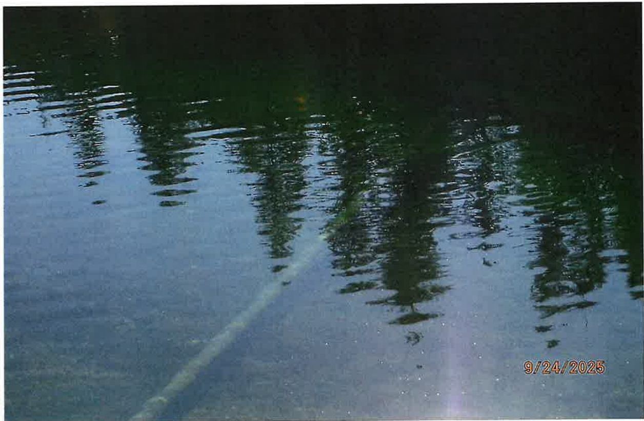
POD – 2-INCH FLEXIBLE SCREENED INTAKE PIPE IN PRIEST LAKE
