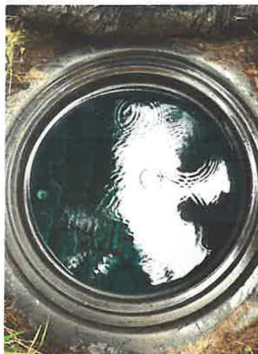
Storage tank with lid open looking into full tank, before burial
