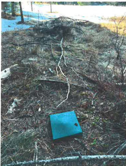
Spring box with buried storage tank in background
