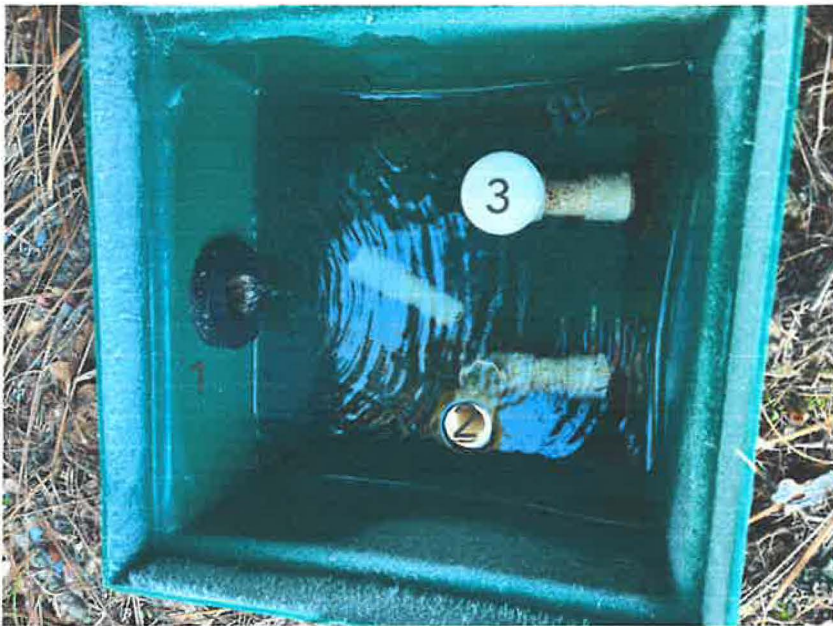
Spring Box: 1- from spring, 2 - overflow, 3 - 1500 gallon storage tank inlet through perforated pipe. Spring flows at an average of 2.4 gallons/min (0.005 cfs)
