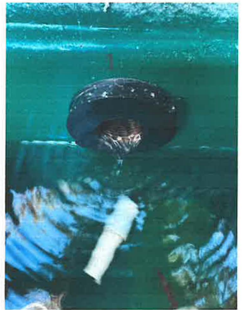
Spring Box: 1- from spring, 2 - overflow, 3 - 1500 gallon storage tank inlet through perforated pipe. Spring flows at an average of 2.4 gallons/min (0.005 cfs)
