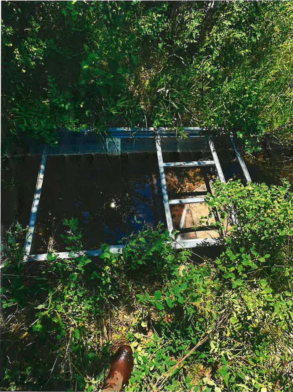
Measuring device suitable for measuring the entire flow of water being diverted in connection with this right.
