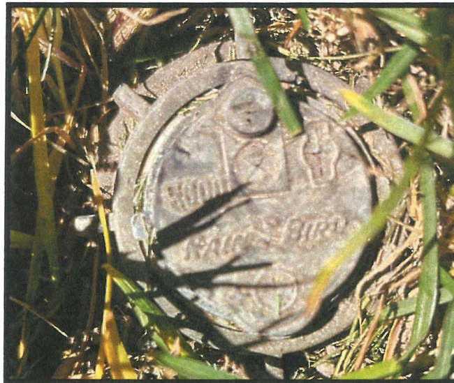
Photo 14- Rain Bird 5000 series rotary heads found in the lawn surrounding the home.
