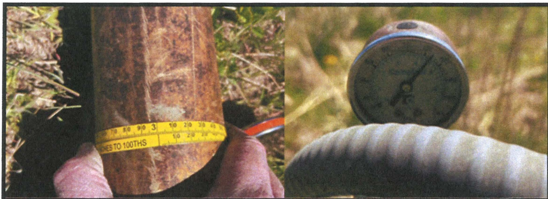
Photos 23 & 24- Diameter measurement of handline (3" aluminum). Pressure gauge on well head while running (64psi).
