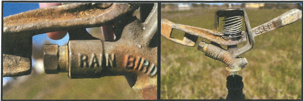
Photos 20a & 20b- Rain Bird sprinkler head on the hand line with 9/64 tip.
