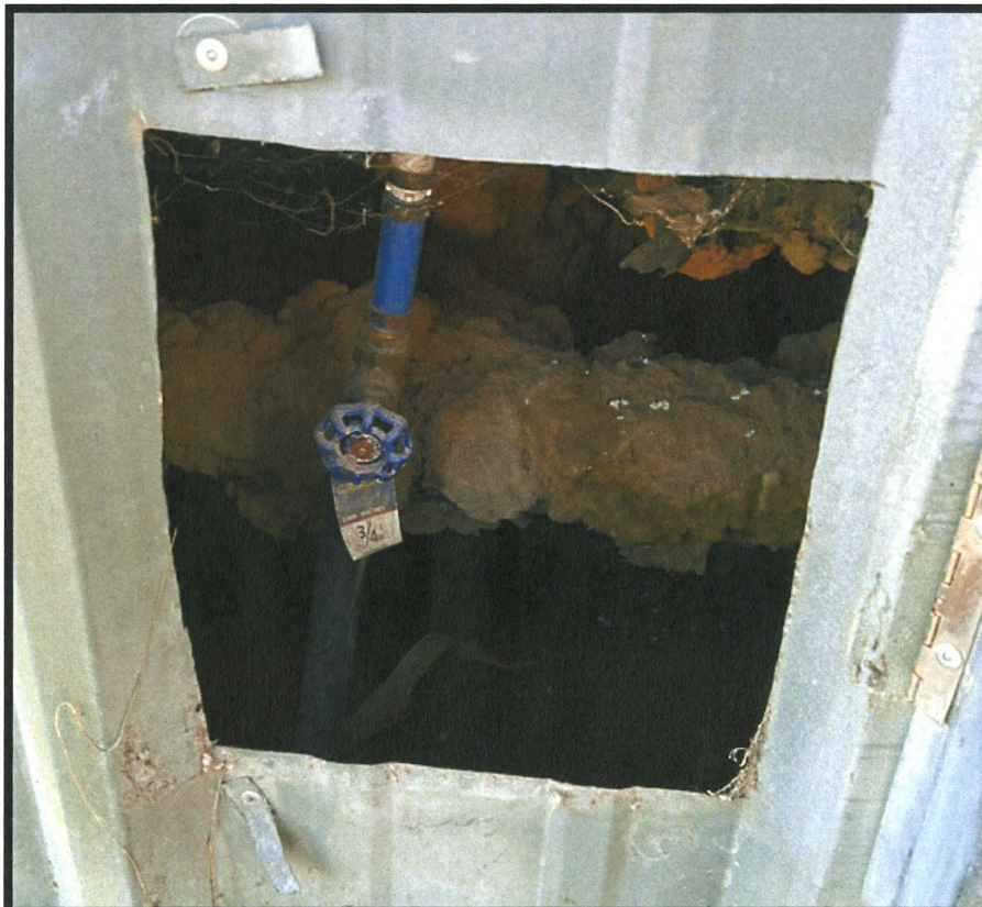
Photo 17 & 18- (above and below) Service hatch for water line into home. The line is reduced to \frac{3}{4} " at the valve.
