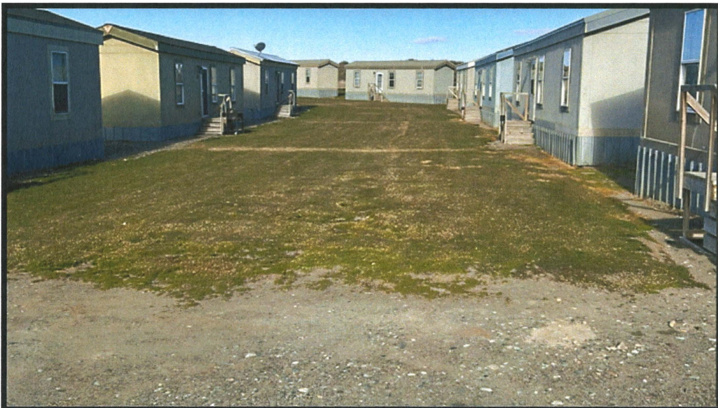
Photo 11- At the SE end facing NW.
