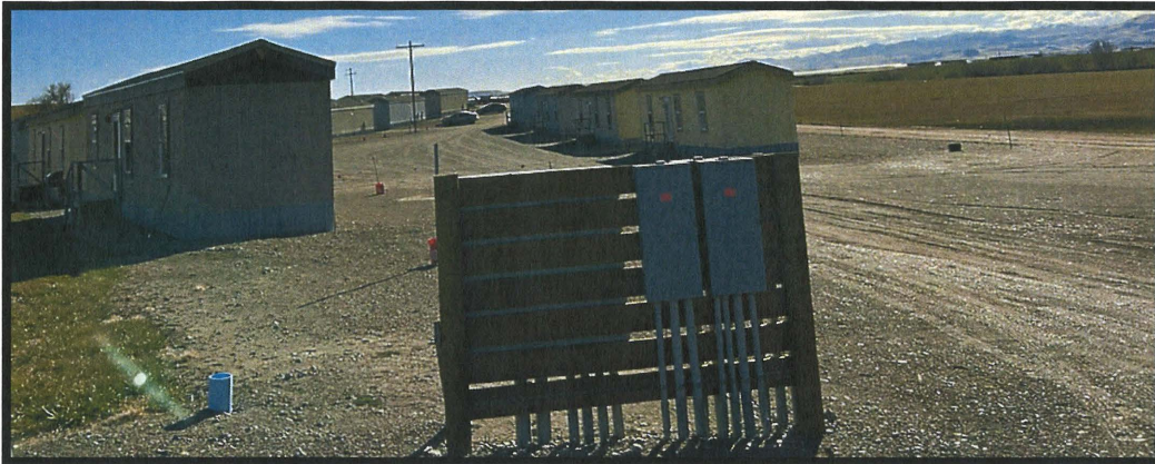
Photo 9- Facing SE- The 4 homes at the SW extent of the development.
