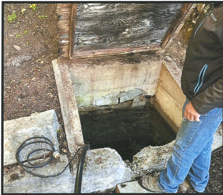
Photo 6- Springbox located to the west of the garden and northwest of the home. Black poly line entering the lower left corner is the diversion line for WR 74-16009 for domestic and stockwater use.
