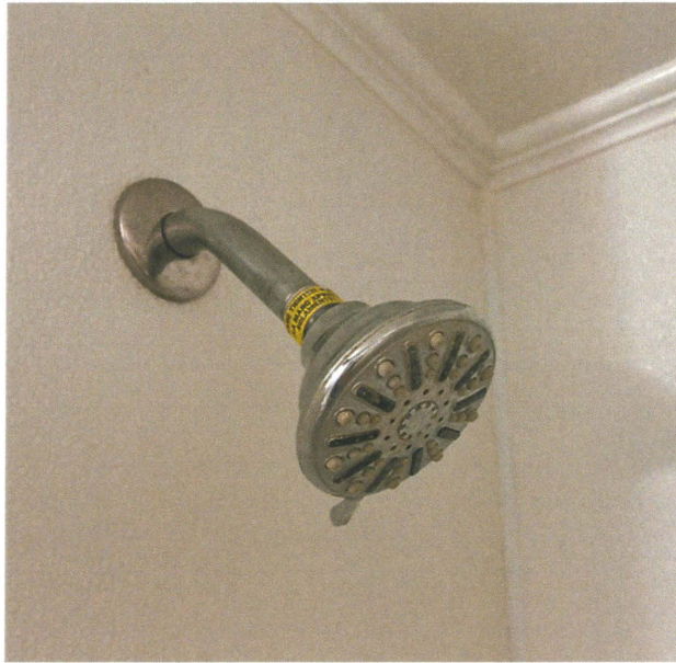
Figure 8 Motel restroom showerhead.
