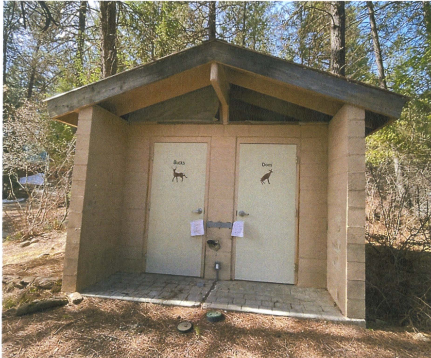
Figure 13 Golf course restroom including two toilets and two sinks.
