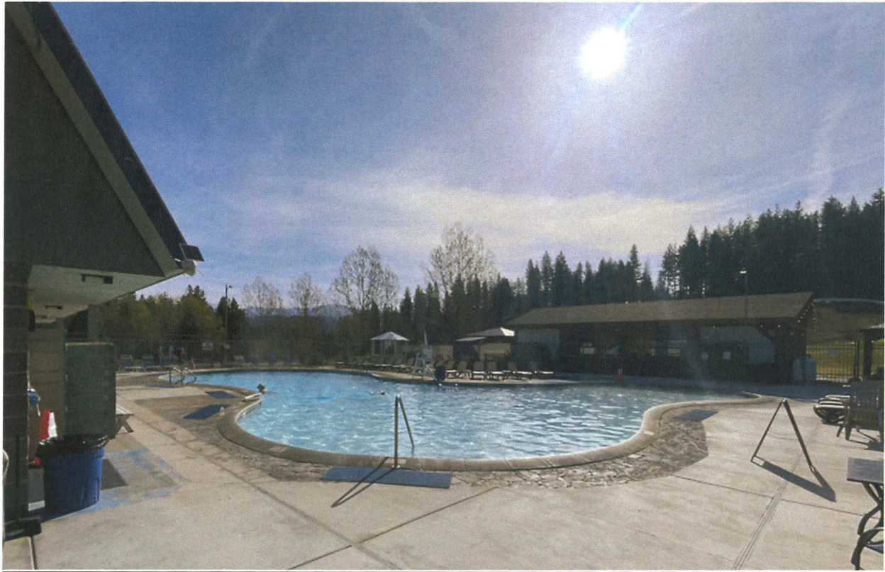
Figure 4 TLRR pool that utilizes geothermal and cold well water.
