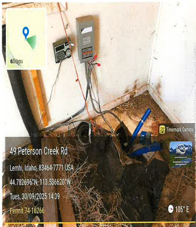
Well Pump House
