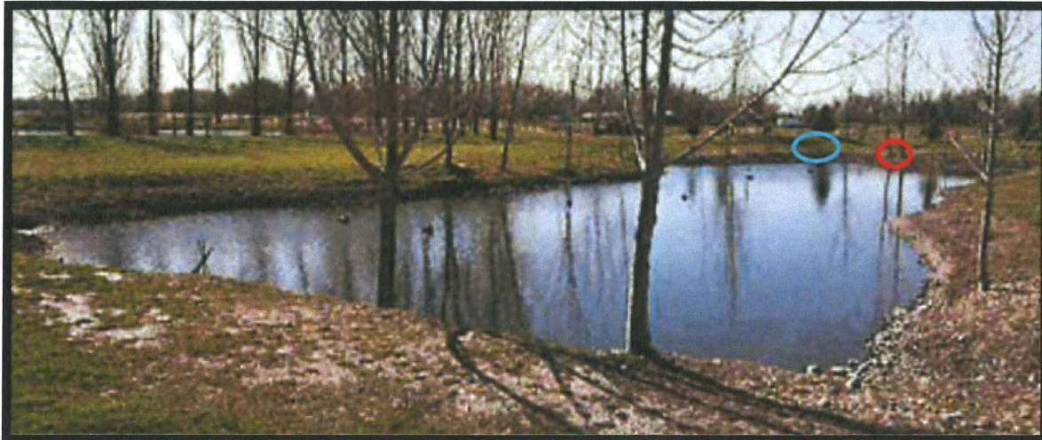
Photo 3- Standing northwest of the pond. The waterfall discharge (circled in blue) and the float sensor (circled in red) are on the south shore of the pond.
