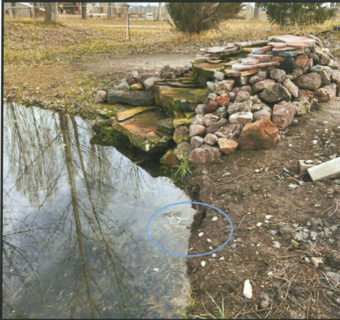
Photo 5- Waterfall with 2" black plastic discharge bypass pipe visible submerged at the shore.
