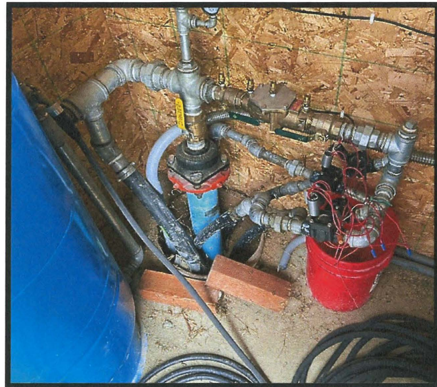
Photos 3 & 4- (Left and right respectively) View through pump house door of pressure tank and manifold. A 2" main is distributed from the manifold into 4- 1 ½ inch poly lines diverting water to the 3 homes and a swimming pool.
