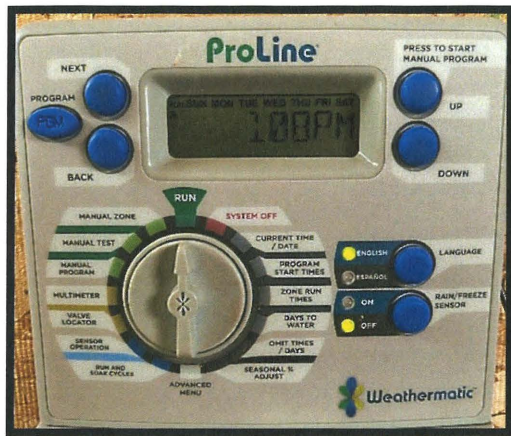
Photo 9-(Left) Controller in pumphouse for front Island irrigation with 4 zones, driplines for trees and small umbrella popups for small bushes in landscaped beds. Photo 10 -(Right) Controller in garage for irrigation surrounding home.
