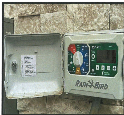
Photo 10 -(Left) Controller for irrigation surrounding home in garage. Photo 11. (Right) Table of zones taped inside the cover for the controller -16 zones with the largest in the southeast (6 rotary heads).
