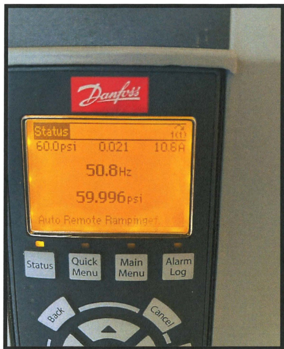
Photo 5 & 6- VLT (variable speed motor control) Control panel (Left) set to maintain 60 PSI in the system. Operation manual (Right) for the controller found in the pump house.
