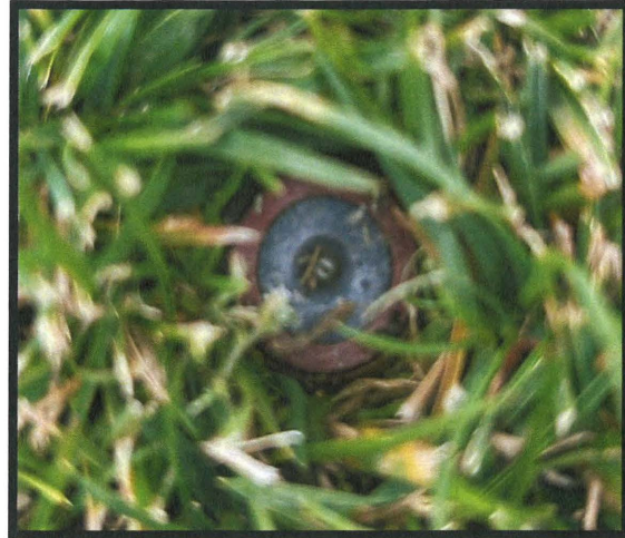
Photo 12 (Left) Rainbird 5000 series rotary sprinklers found through out larger areas. Photo 13 (Right) Small umbrella pop up sprinklers found in areas bordering structures and in landscaped beds.
