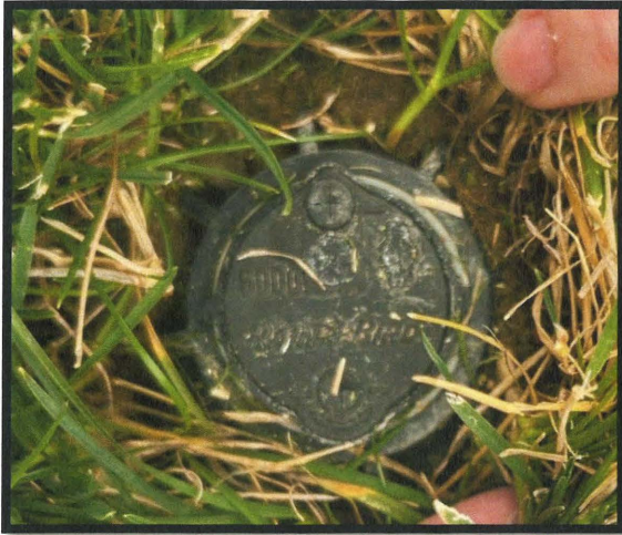
Photo 12 (Left) Rainbird 5000 series rotary sprinklers found through out larger areas. Photo 13 (Right) Small umbrella pop up sprinklers found in areas bordering structures and in landscaped beds.
