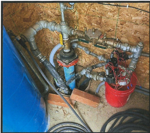
Photos 3 & 4- (Left and right respectively) View through pump house door of pressure tank and manifold. A 2" main is distributed from the manifold into 4- 1 1/2 inch poly lines diverting water to the 3 homes and a swimming pool.
