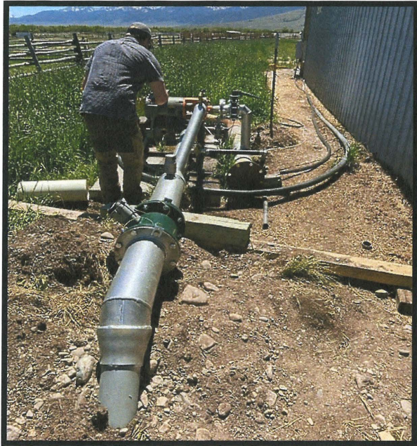
Photo 4-(upper left) Pump station with 2- 10Hp centrifugal pumps stacked with flowmeter at green flange.
