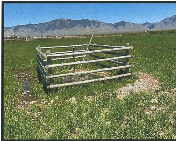
Photo 2-(left) Enclosure surrounding bubbler (intake) located north about 50 yards north of the headgates on west side of wastewater ditch. Photo 3-(right) Bubbler with large screen overtop of 12" vertical pipe.
