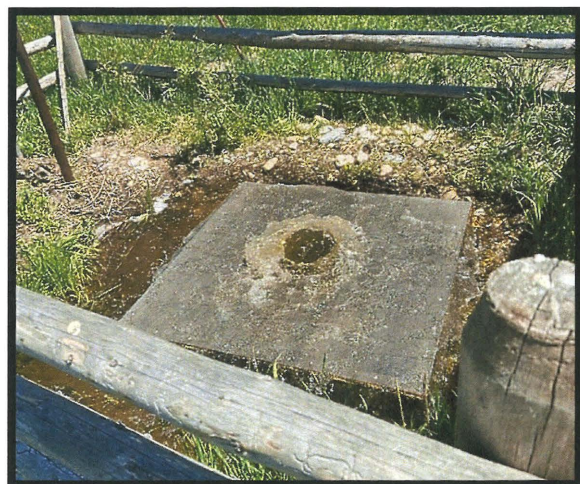
Photo 2-(left) Enclosure surrounding bubbler (intake) located north about 50 yards north of the headgates on west side of wastewater ditch. Photo 3-(right) Bubbler with large screen overtop of 12" vertical pipe.
