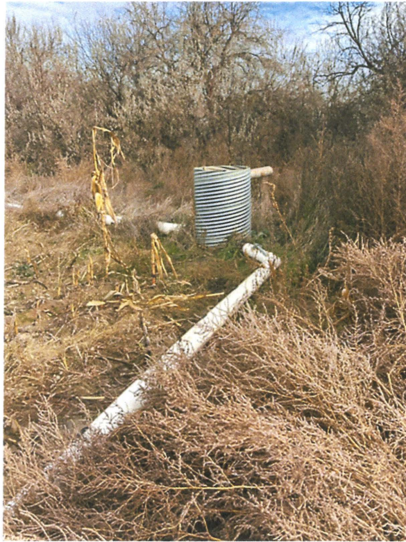
Figure 13 Riser associated with field 2.
