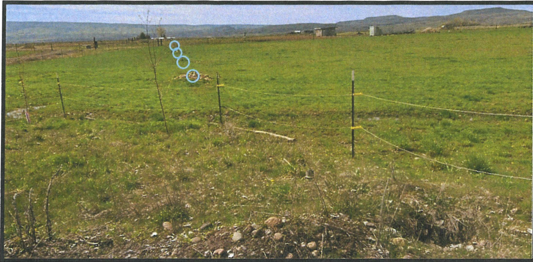
Photo 12- Facing south-A row of 4" PVC risers (circled in blue) located in the southeast extent of the POU.
