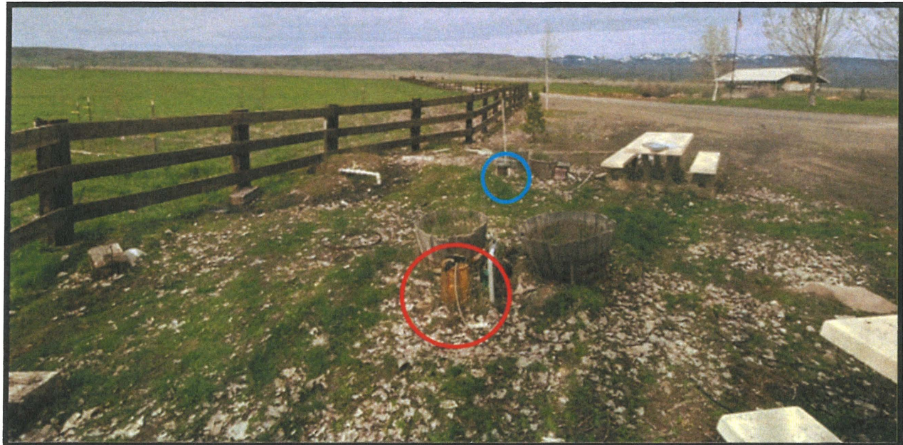
Photo 3- Facing west the irrigation well head is circled in red and the domestic well head is circled in blue.
