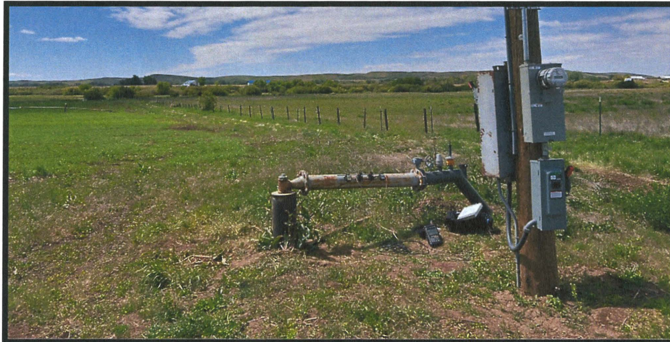
Photo 1– Standing in the northwest corner facing south. The row of risers run on the near side of the fence line.
