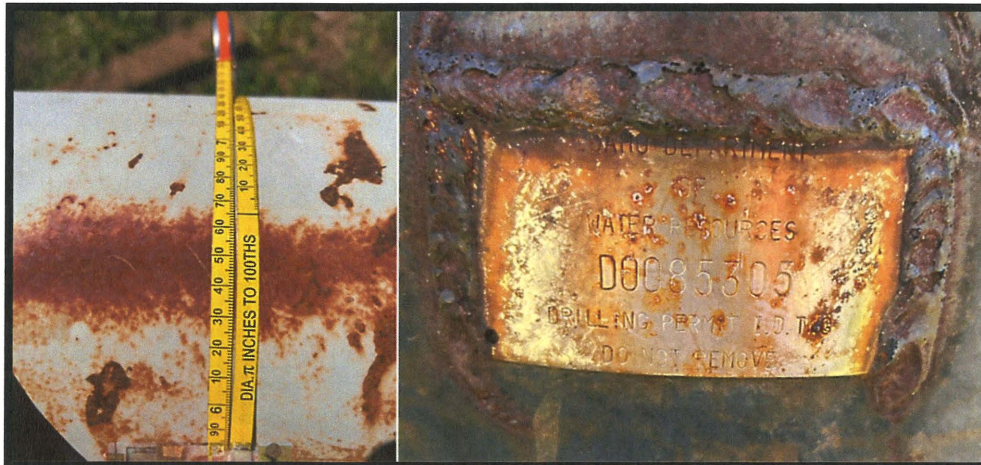
Photos 2 & 3 – Diameter measurement of the steel main (left), Well head tag (right).
