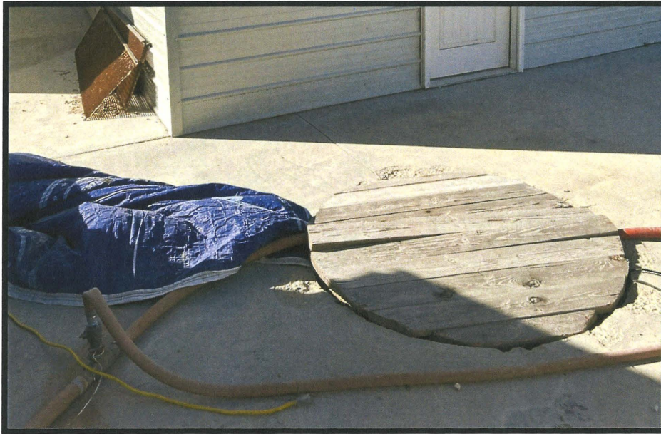
Photos 15 & 16- Valve box located north of the pump house. The galvanized line to the batch tower and the 2" flex line to the truck wash can be seen in the lower image. An additional hose is attached to the manifold for cleanup under the batch tower.
