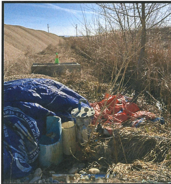
Photos 2 & 3- Well head in the southwest corner of the POU. A pipe with a hand valve is welded to the casing allowing for artesian flow to be cracked open to prevent freezing. The well head is also covered with a insulated blanket in the winter to protect it from low temperatures.
