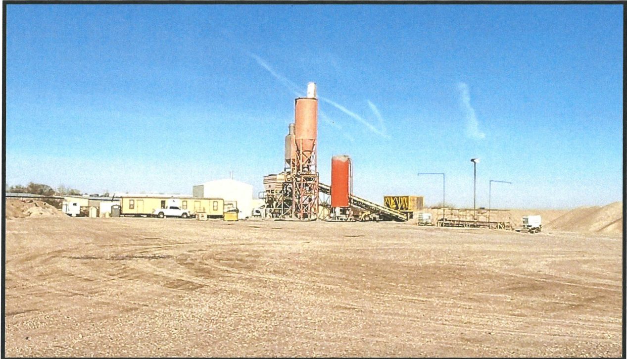
Photo 1- In the southeast corner of the POU facing west. The control room skid, boiler/chiller room, batch plant, and truck wash can be seen in frame from left to right respectively.
