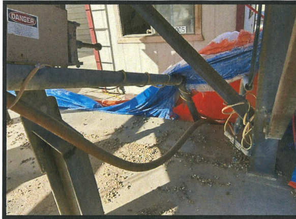
Photo 17- 3" galvanized and 2" flex line ramping up along the frame to the top of the batch tower.
