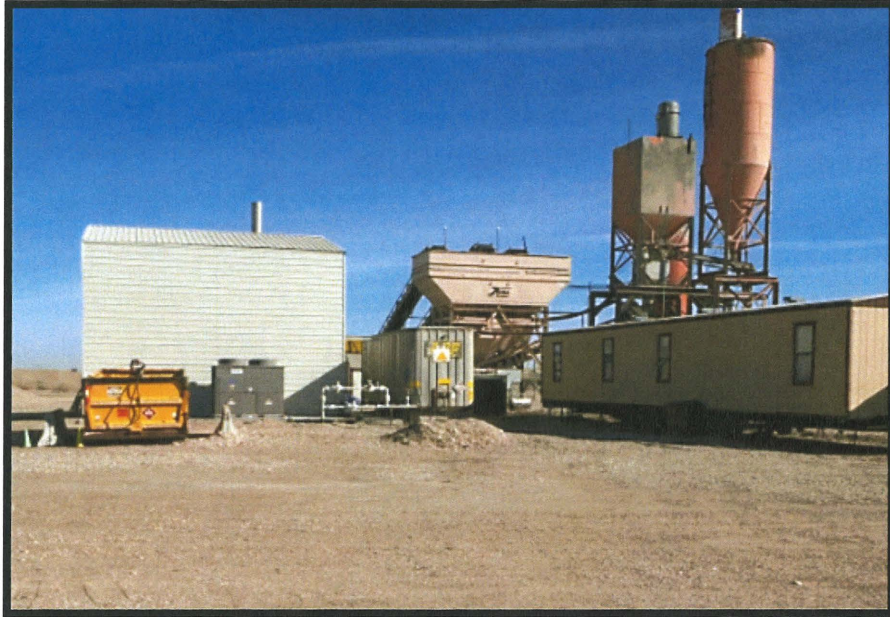
Photo 7- Facing north between the well head and boiler room.
