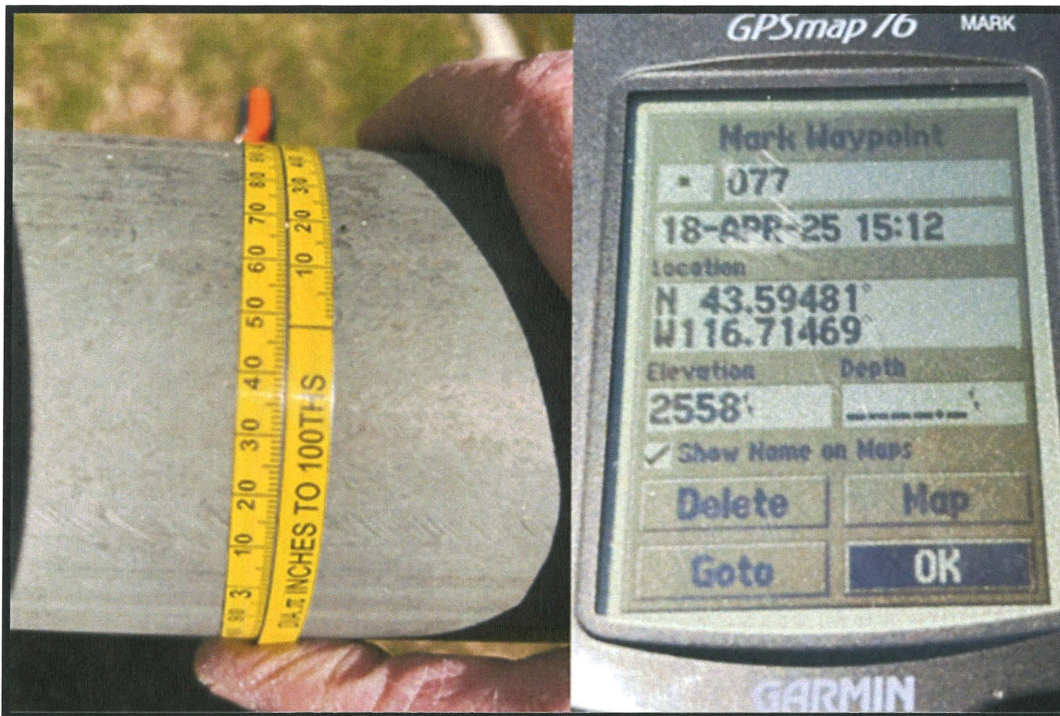
Photos 5 & 6- Steel Mainline diameter measurement and GPS coordinates for irrigation well head.
