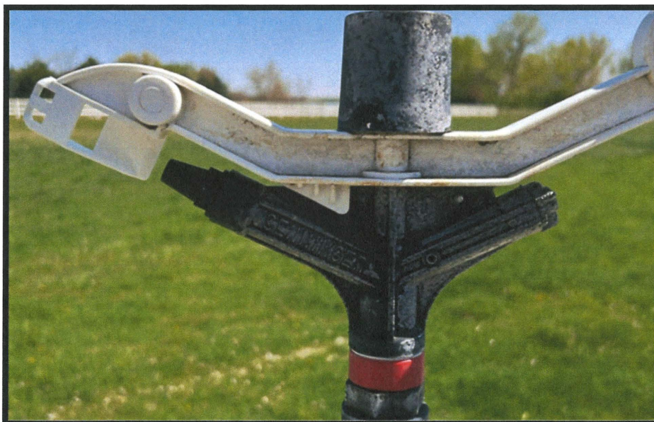
Photo 12- ¾" Senninger Impact Sprinklers found through out field sprinkler system with cup enclosed popups in the middle two rows.
