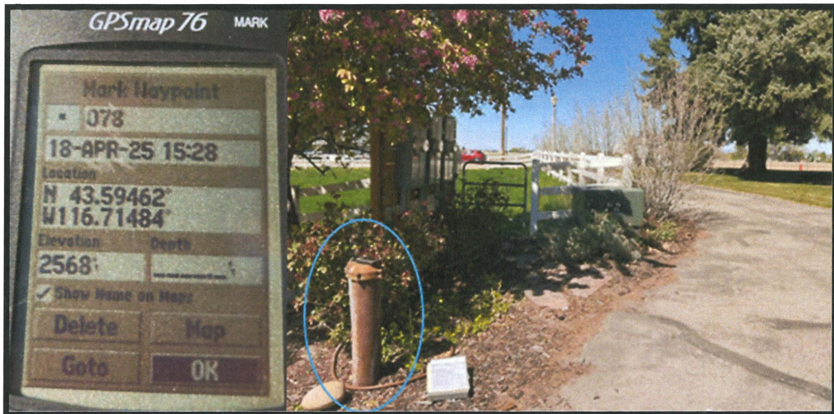
Photos 16 & 17- GPS Coordinates for the domestic/stockwater well head circled in blue.
