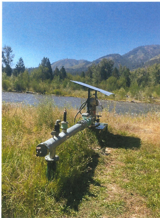
Figure 3 Point of diversion for right 65-23671 for irrigation from South Fork Payette River.
