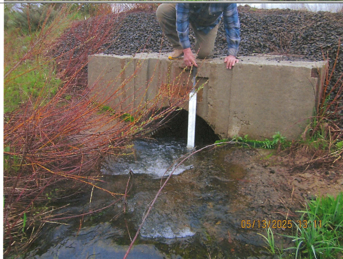
Figure 2. Water flowing out of The Lake Wilderness Ranch Reservoir through a culvert under Old Dry Buck Road.
