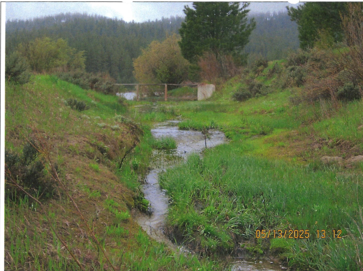
Figure 1. Water flowing out of The Lake Wilderness Ranch Reservoir.
